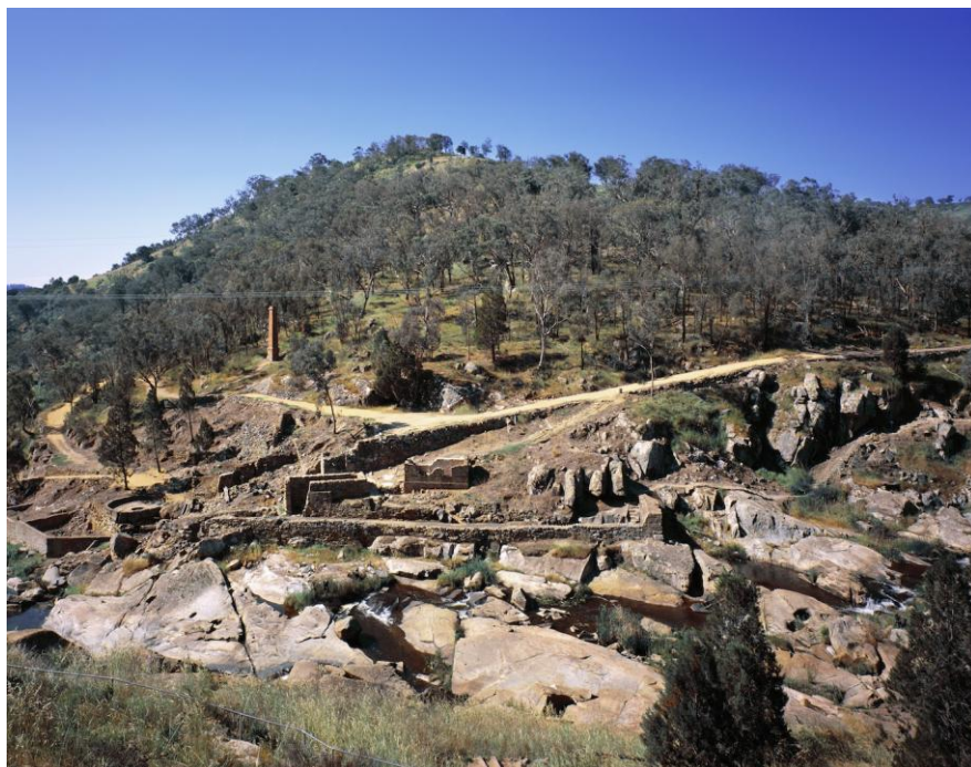
Reefer Battery ruins Adelong Creek
