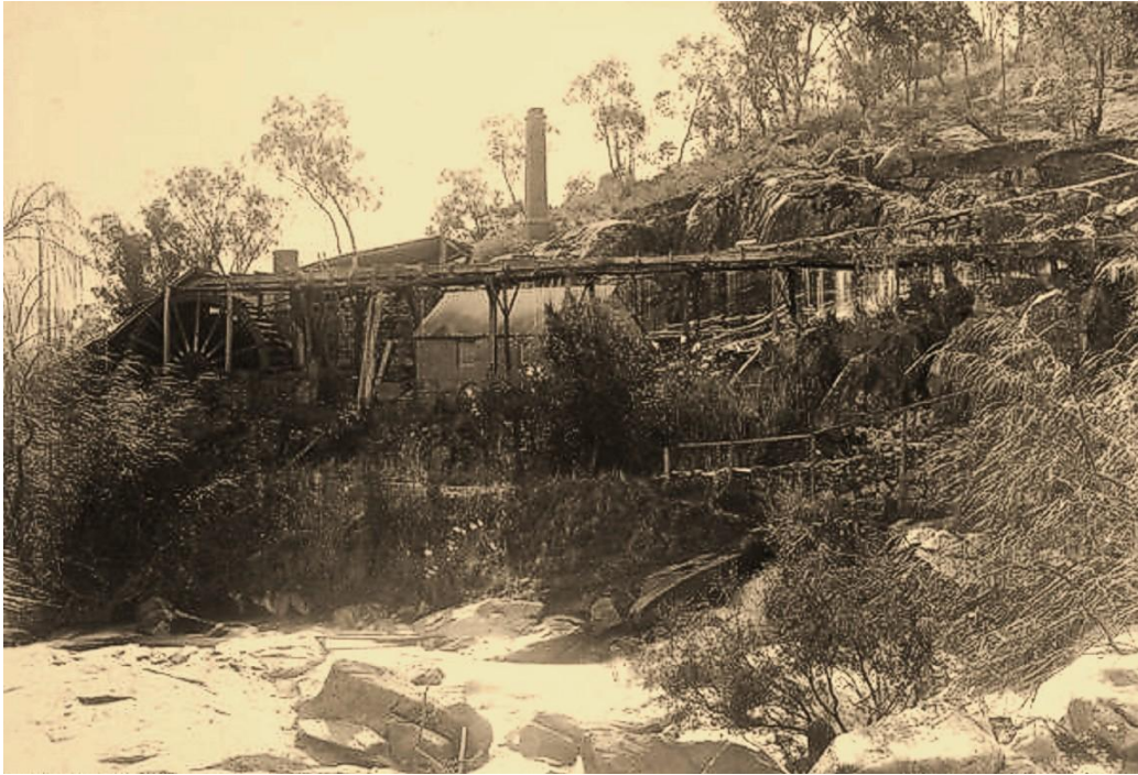
The Reefer Battery showing the upper water wheel, flume, office, reverbatory furnace stack c 1915 R C Strangman, NLA.
