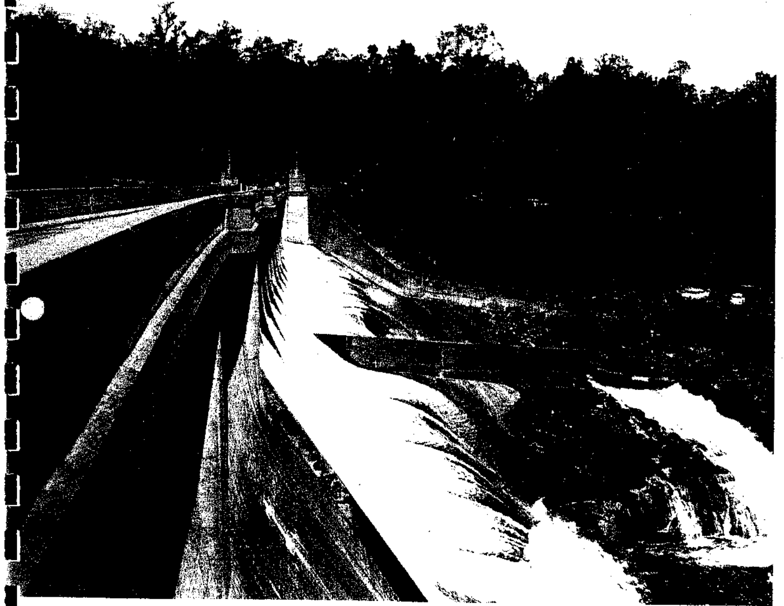
Canning Dam overflowing in 1974.
