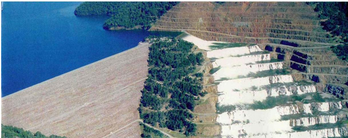
**Figure 5 Dartmouth Dam during spilling down the quarry benches**
