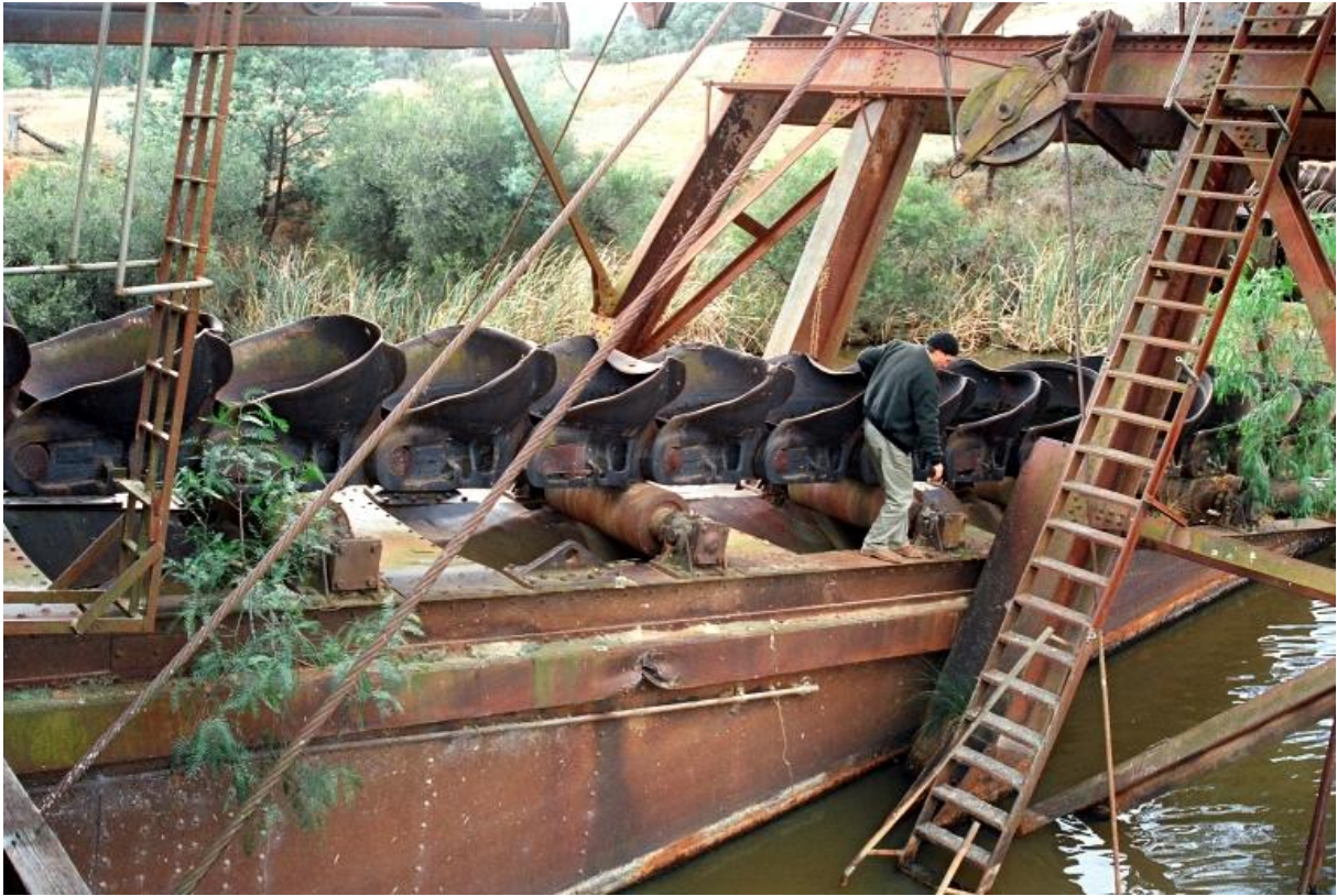
Figure 8: Forward end of the bucket ladder, near the submerged tip. Viewed from SW, with a Park Ranger for scale. The bucket band sits on rollers on the top face of the bucket ladder, and here passes between legs of the fore-gantry. The bottom tumbler and lower buckets are submerged. (Photo by C. Doring 1994.)
