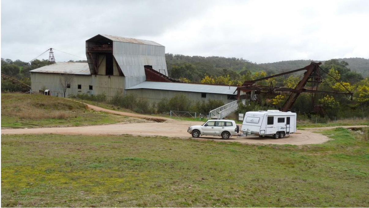
Figure 1: Eldorado Dredge viewed from SE, partly obscured by trees and by the earthen banks of its pond. Bow end with bucket ladder and fore-gantry at right, superstructure at centre, stern with discharge chutes at left. (Photo by Phelan, from the Web.)
