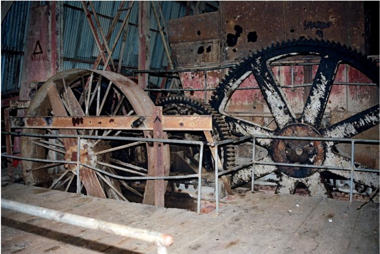
Figure 9: Large gears (right and centre) driving the top tumbler (hidden) that drove the bucket band. These are next to the top of the bucket ladder (also hidden), set high in the central superstructure. Power came from a large electric motor on the deck far below, via a flat belt onto the flat-face pulley at left (belt now missing). The waist-high guard railing gives scale. (Photo by C. Doring 1994)
