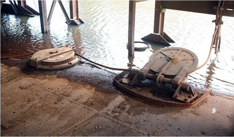
Figure 10: Mooring pulleys on the deck near the stern, starboard side. The left pulley is one of several guiding the exposed cable across the deck from the winch to here. Cable from the right-hand pulley goes to an anchor point on land, and the pulley swivels to accommodate variations in anchor height.
