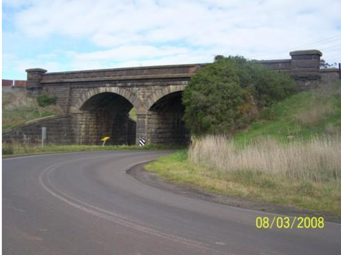
Cowies Creek Bridge No.1 across Bluestone Bridge Road, 2008.
