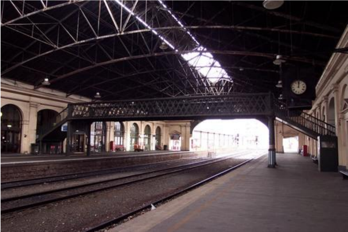
Inside the train shed at Ballarat Railway Station with the footbridge in the centre.
