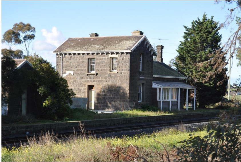
Moorabool Railway Station, now a private dwelling, 2010
