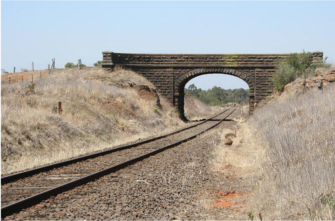
Lethbridge bluestone overbridge
