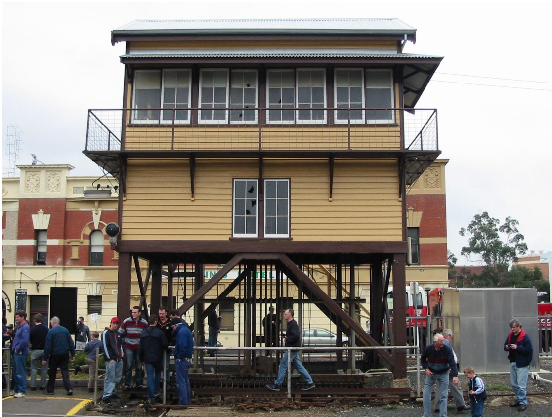
The main signal box at Ballarat east of the Railway Station.
