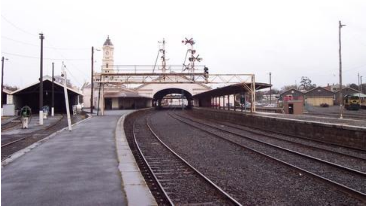
Ballarat Railway Station from the east with the train shed in the centre and the clocktower behind.
