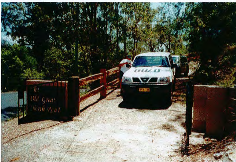
Clockwise from top left: general view downhill before pavement resurfacing; culvert outlet in buttness; buttnessed retaining wall; new entrance gates, and possible plaque position, at bottom of Devines Hill; typical culvert outlet in retaining wall.
