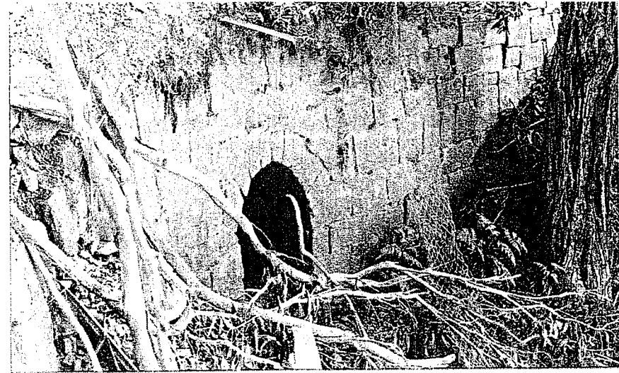
Fig 4: Culvert outlet with arched voussoir stones, set in curved retaining wall; 13.9 km north of Mt Manning junction (1830-31)
