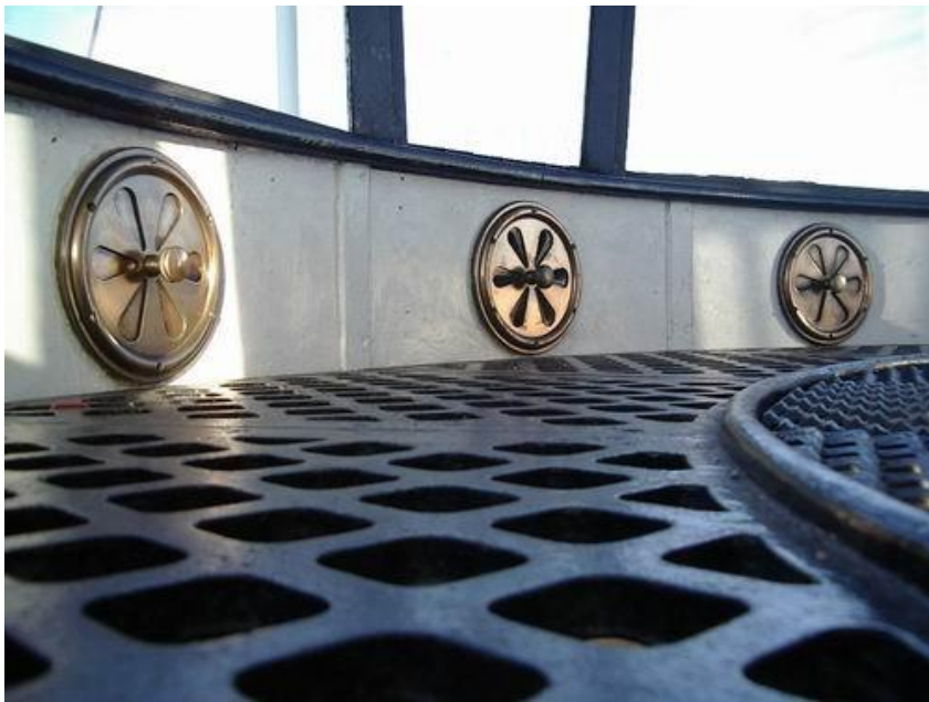
Green Cape lantern house gallery walkway showing ventilators
