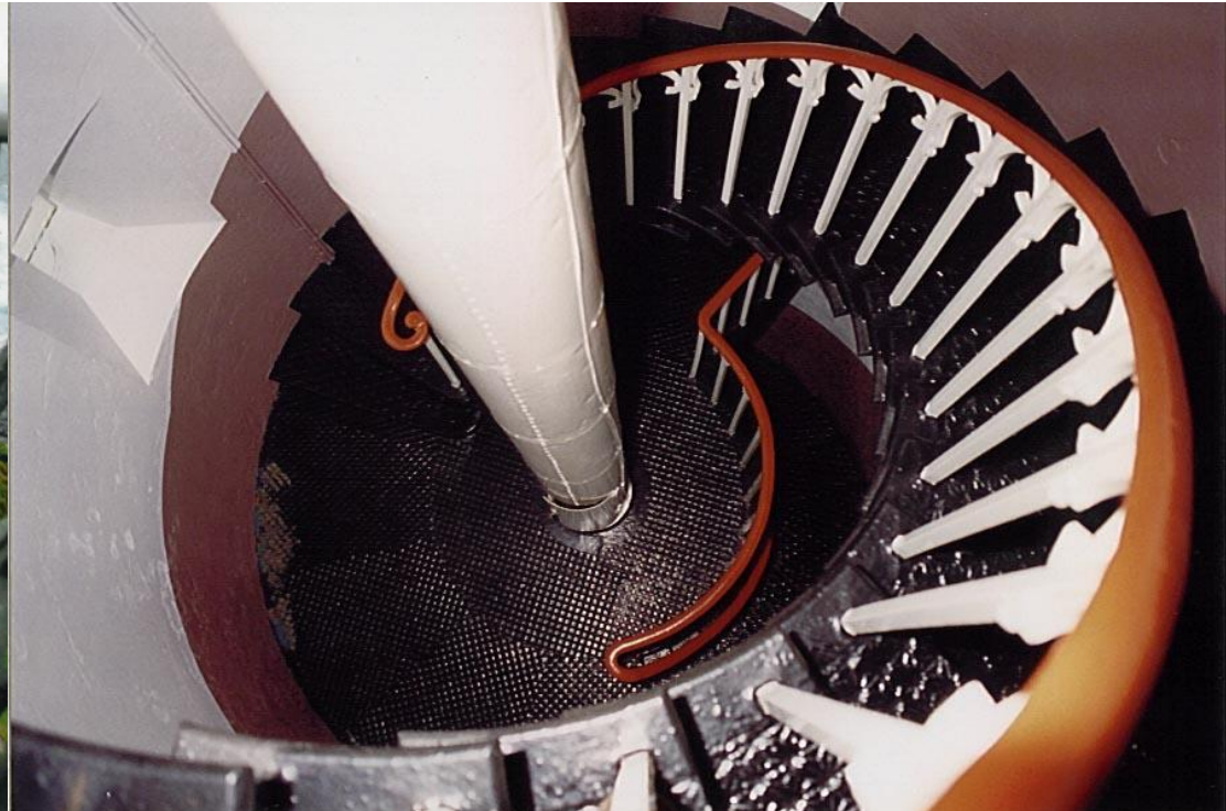
Green Cape Lighthouse Spiral Cast Iron Stairway and Weight Tube
