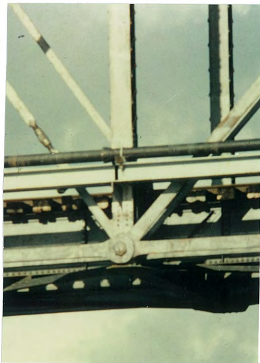
Close up views of some of the pinned joints.
