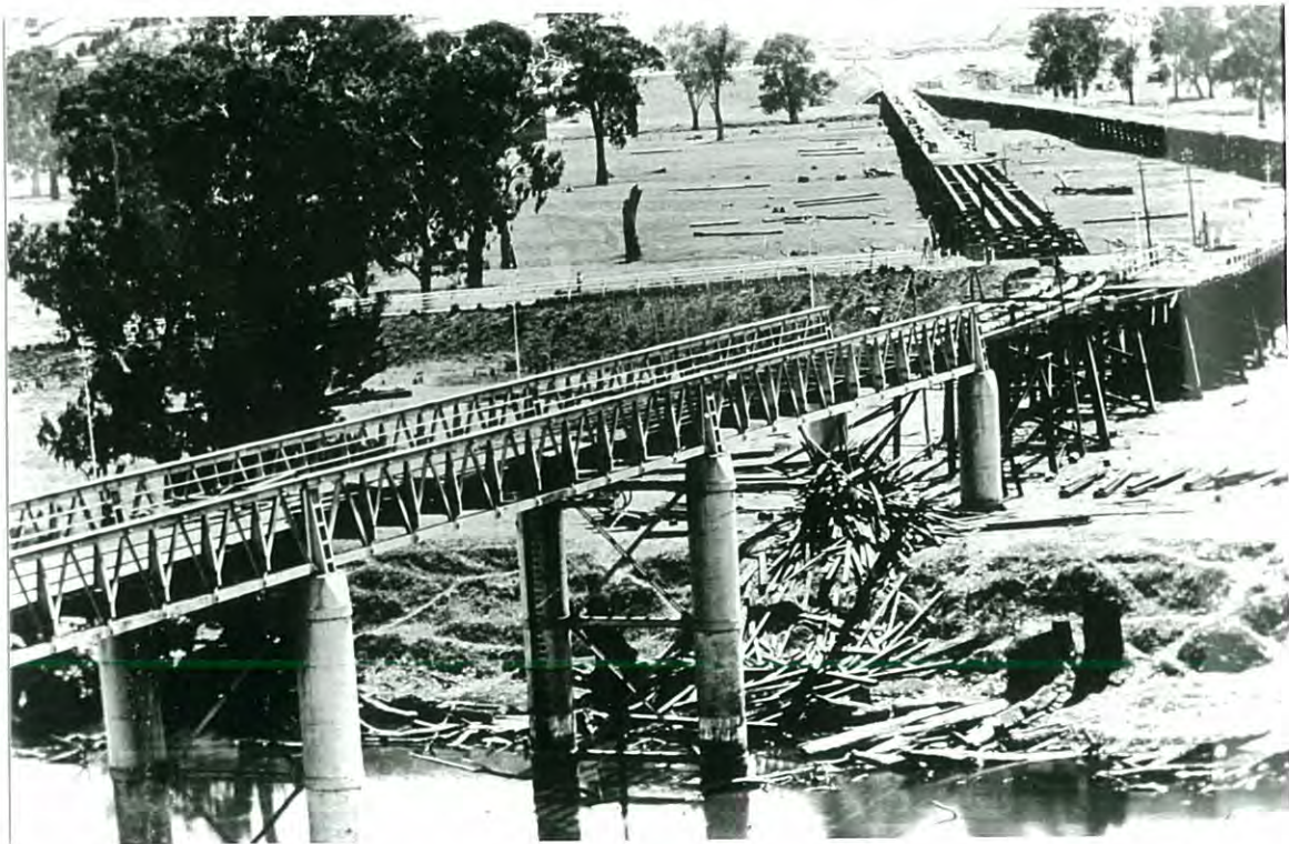
The scene in 1898 looking north as the reconstructed viaduct nears completion. The iron truss Prince Alfred Bridge is in the foreground and the 1869 viaduct is on the far right.
