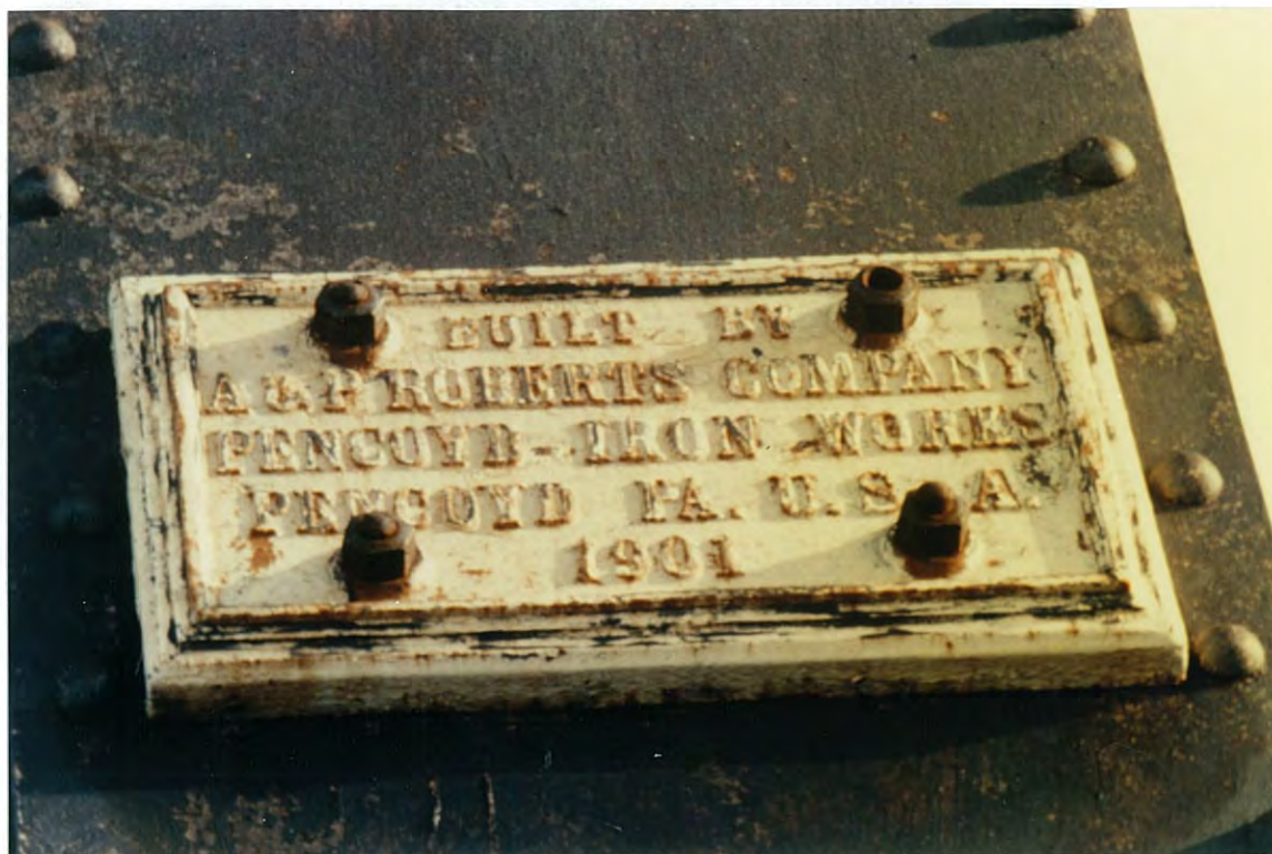
The maker's plate on the steel railway truss at Gundagai.
