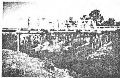
Figure 12 Percy Allan (1861-1930), "Mr Timber Truss Bridge", is synonymous with timber construction. He joined the Public Works Department in 1878 and became a competent and innovative bridge designer. Probably his best known bridges are the electrically operated swing spans at Pyrmont and Glebe Island. His 1894 designs of the pony truss (above) and overhead-braced trusses (right) bear his name.
