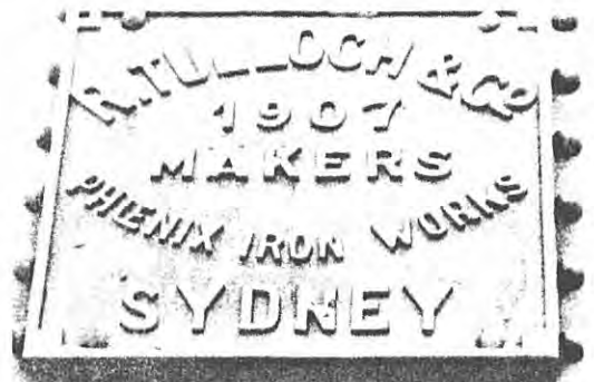
Figure 18 Makers plate on the 1907 railway trusses over the Nepean River, Penrith.
