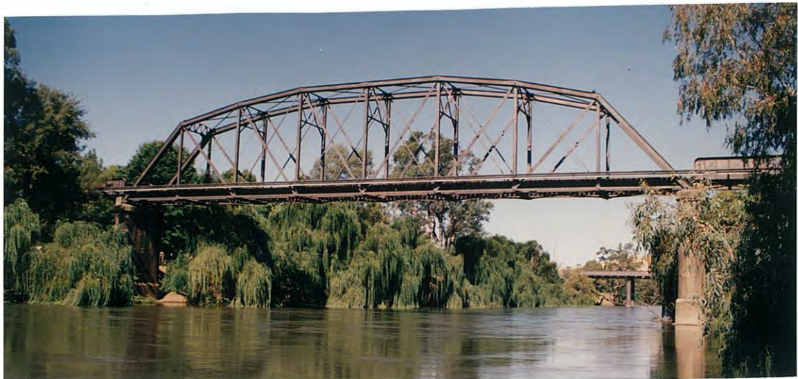
Top the 1867 Prince Alfred Bridge and below the 1903 railway truss.
