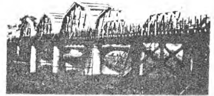
Figure 11 J.A. McDonald redesigned the OLD PWD truss to carry much heavier loads (top left) and the new truss (left) bears his name. An important feature was the inclusion of opposing steel wedges (above) to "tighten-up" the bridge. His largest project was the 1893 Cowra Bridge (right) for which he designed three 49m (160 feet) composite overhead-braced trusses.
