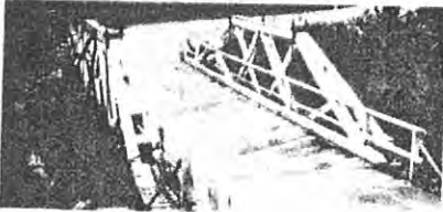
Figure 11 J.A. McDonald redesigned the OLD PWD truss to carry much heavier loads (top left) and the new truss (left) bears his name. An important feature was the inclusion of opposing steel wedges (above) to "tighten-up" the bridge. His largest project was the 1893 Cowra Bridge (right) for which he designed three 49m (160 feet) composite overhead-braced trusses.
