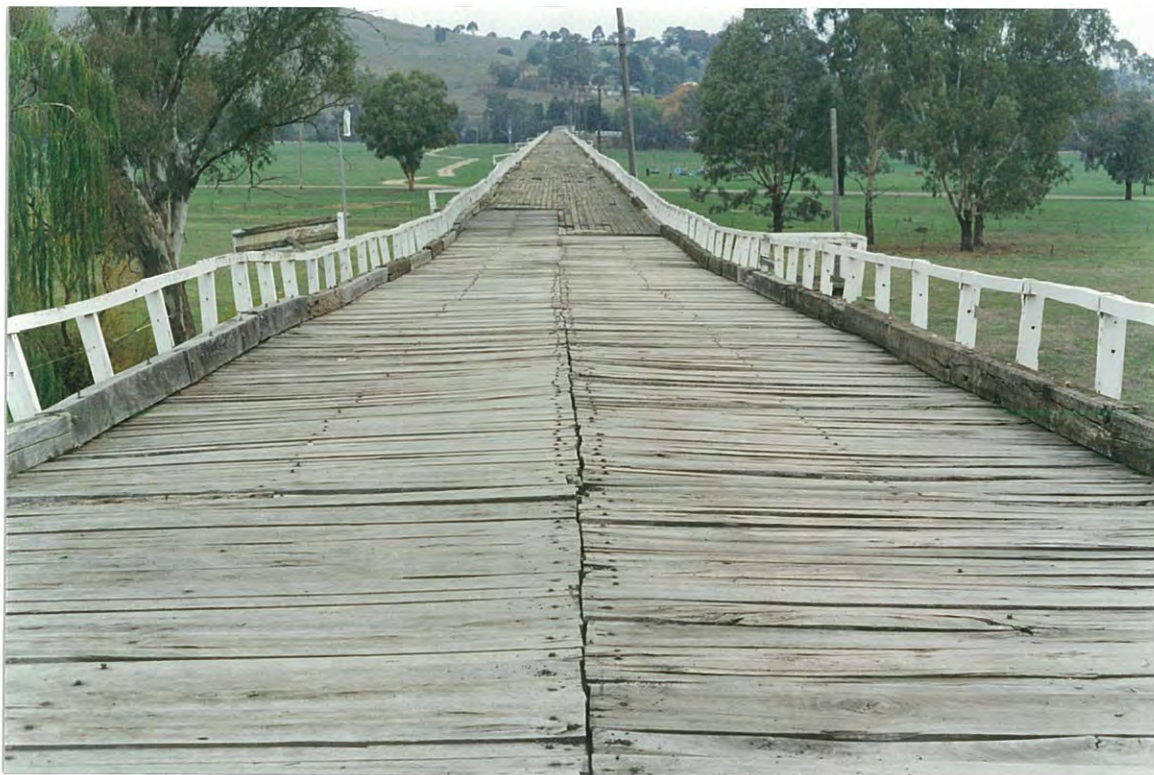
Deck repairs undertaken during the early 1990s.
