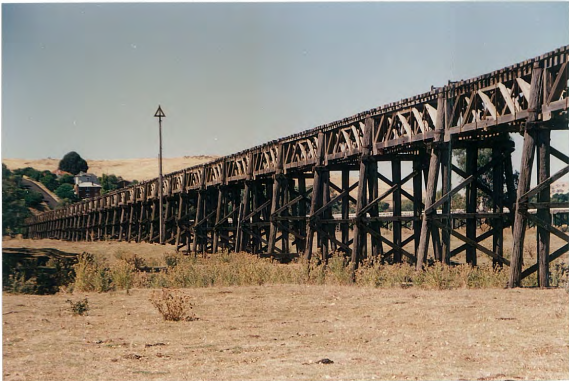
Top A typical timber truss span of the railway viaduct, revealing its details and showing its dominance over the timber beam road viaduct and below the high-level railway viaduct "marching" across the flood plain.
