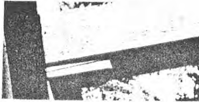
Figure 11 J.A. McDonald redesigned the OLD PWD truss to carry much heavier loads (top left) and the new truss (left) bears his name. An important feature was the inclusion of opposing steel wedges (above) to "tighten-up" the bridge. His largest project was the 1893 Cowra Bridge (right) for which he designed three 49m (160 feet) composite overhead-braced trusses.
