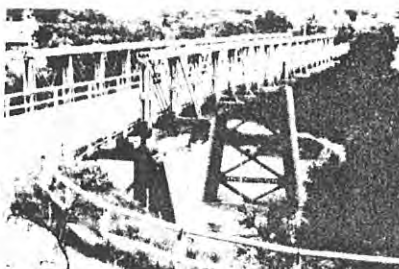
Figure 14 Two of DeBurgh's major bridges. The two-span pony trusses over the MacDonald River at St. Albans, and the deck truss over the Lane Cove River known as the DeBurgh Bridge. There are plans to preserve this historic bridge.
