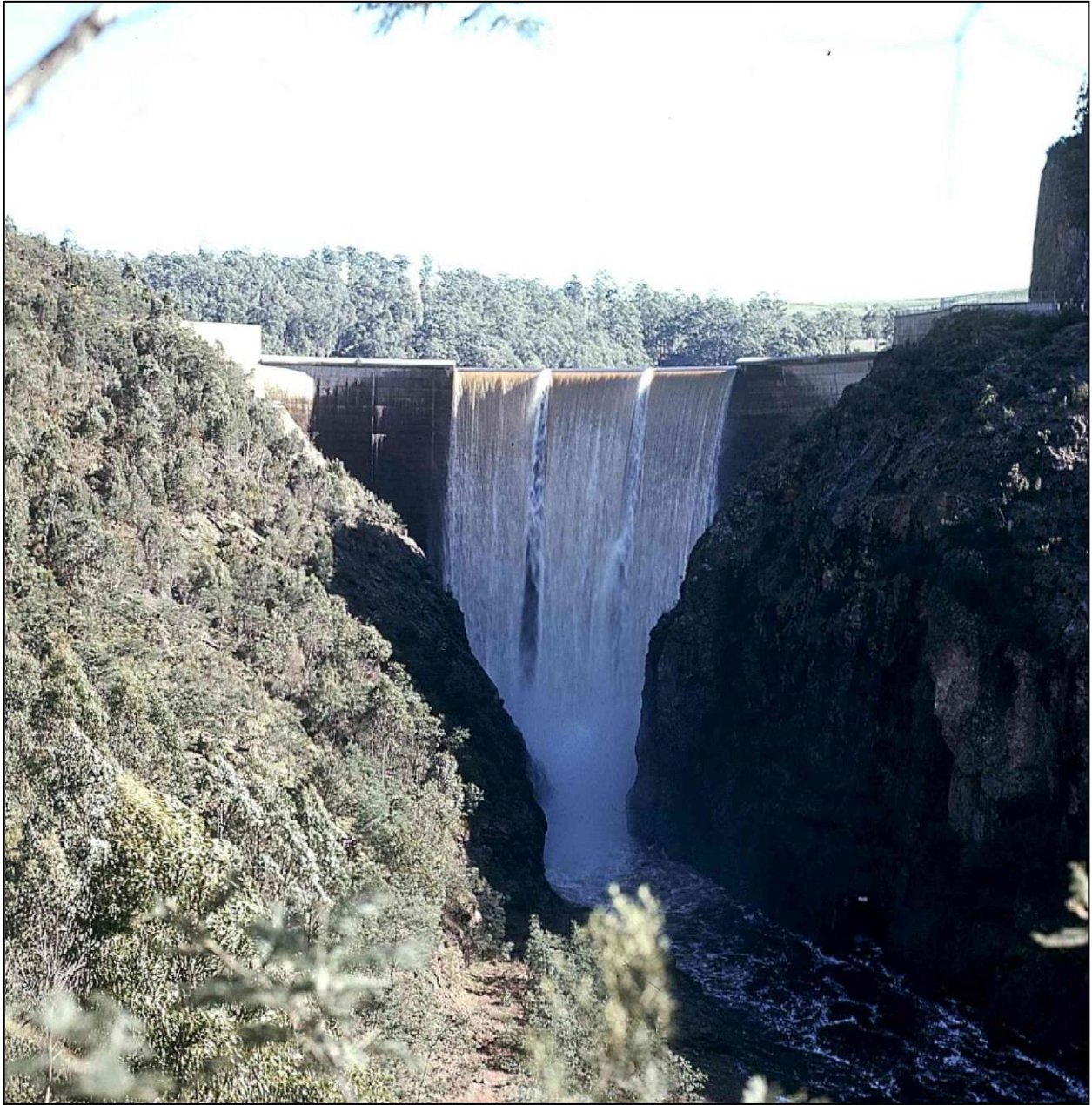
Devils Gate Dam – lower spillway in operation
