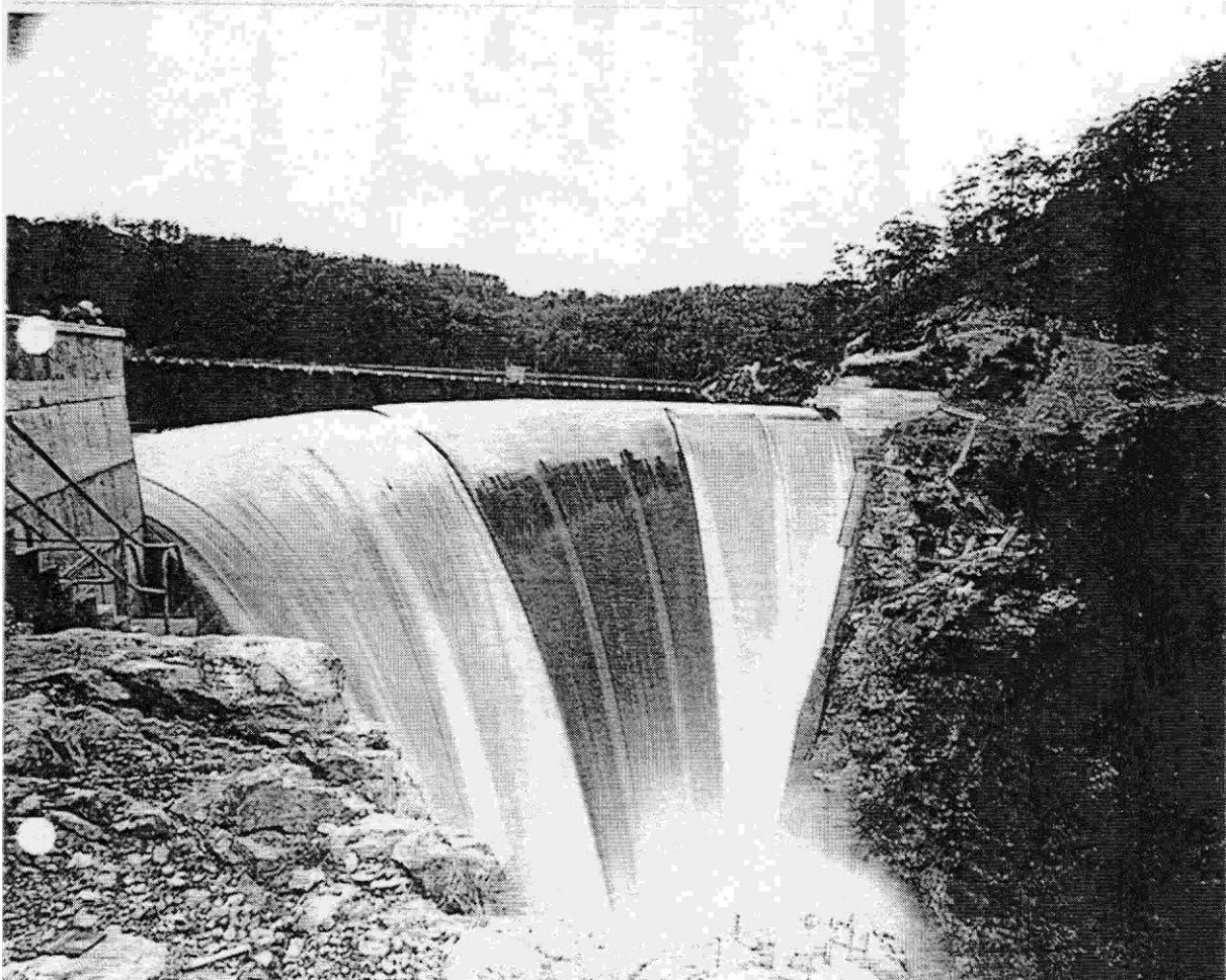
Devils Gate Dam – whole spillway in operation
