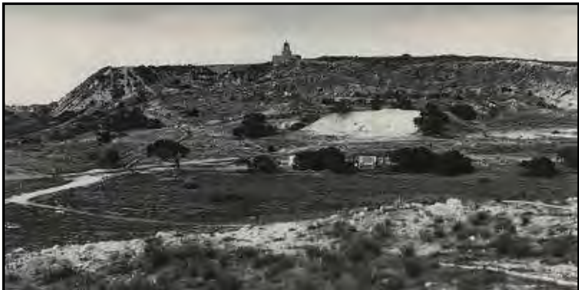
Figure 3. View looking east towards Buckland Hill c. 1942
