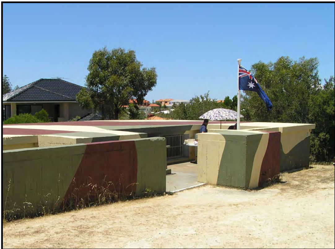
Figure 23. 5.25 inch Gun Command Post
