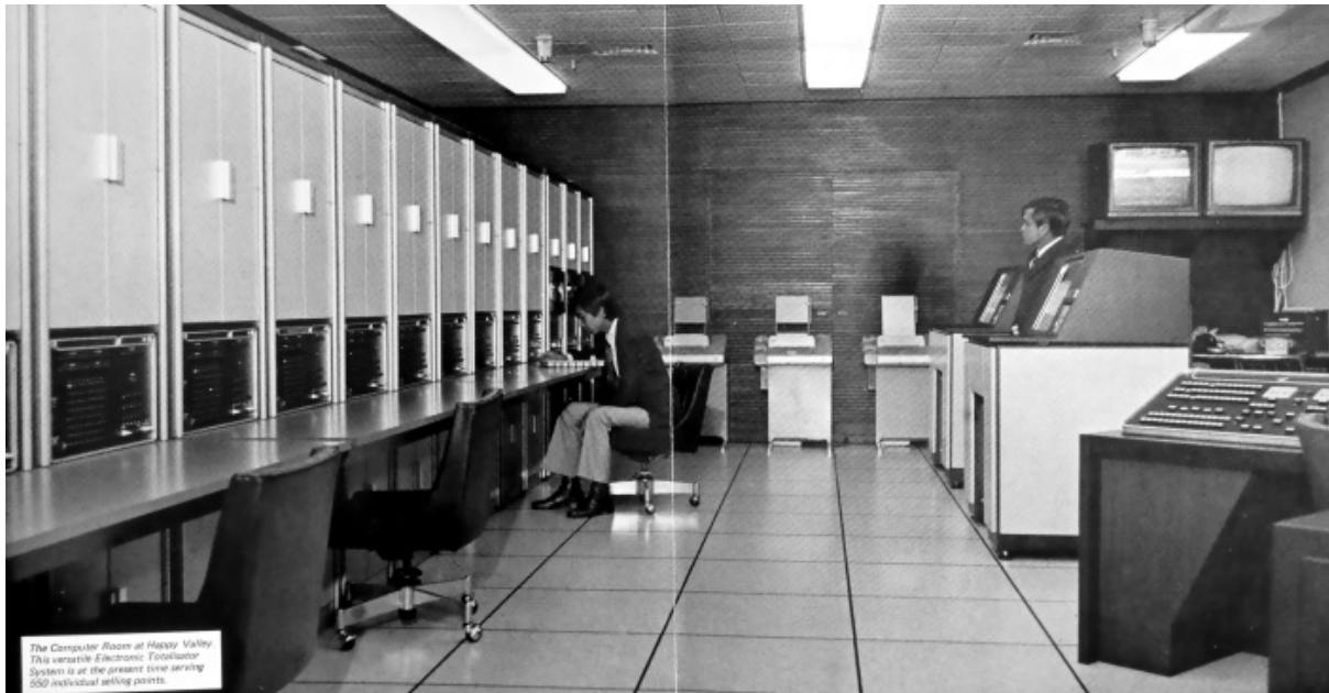
The Hong Kong PDP8 Totalisator System at Happy Valley
