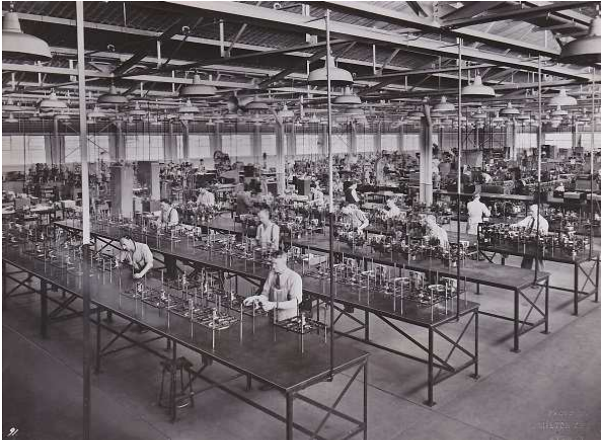
Part of the Assembly Section
