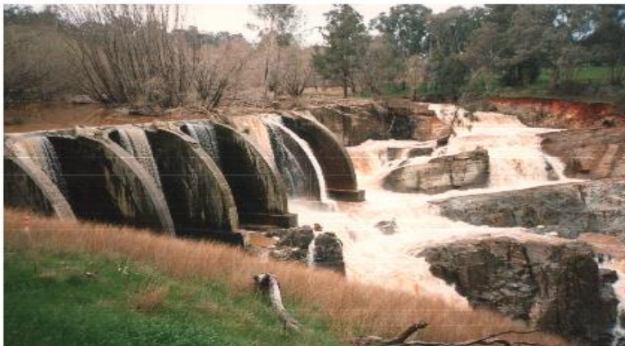
Junction Reefs Dam during recent flooding. Image: NSW Dams Safety Committee.
