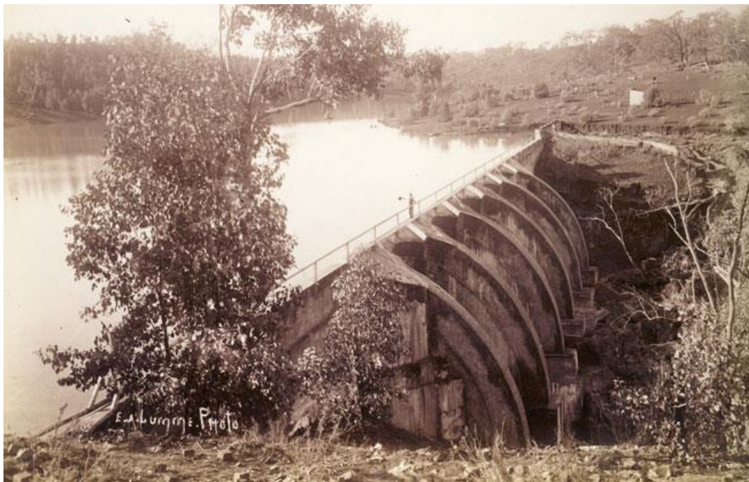
Junction Reefs Dam shortly after construction. Image: E A Lumme.
