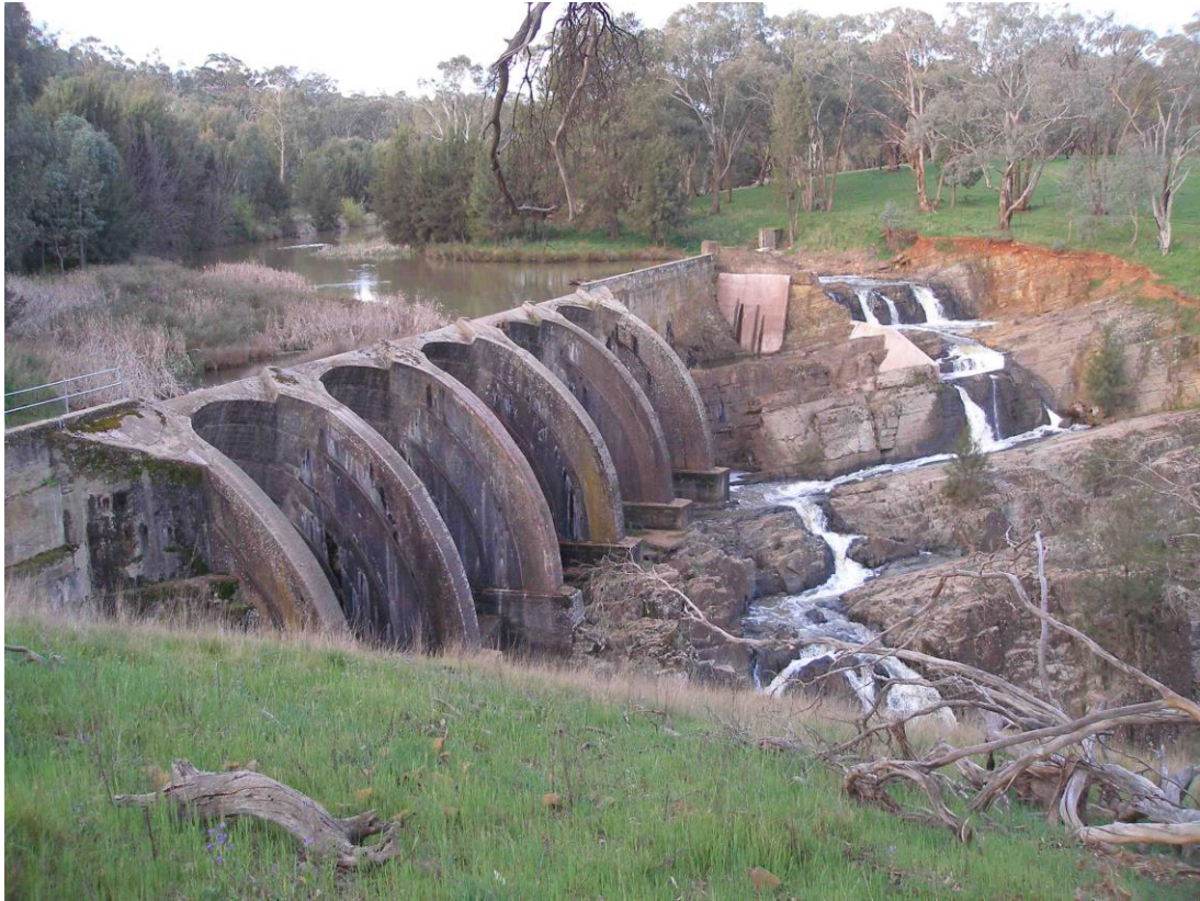
Junction Reefs Dam, September 2009. Image: Source unknown.
