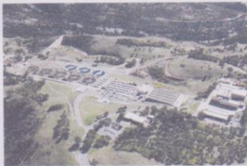
above and top: Lower Molonglo Water Quality Control Centre
