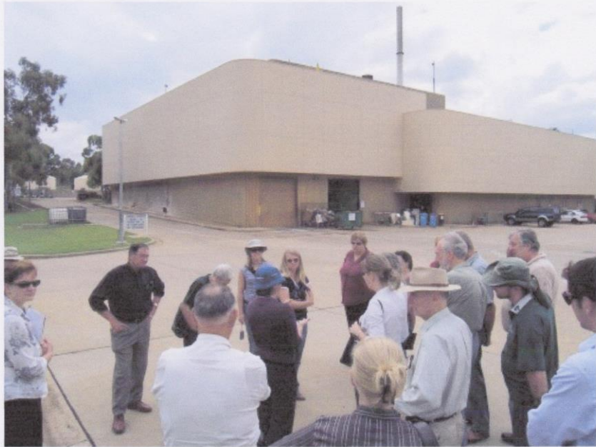
Incinerator at the LMWQCC
