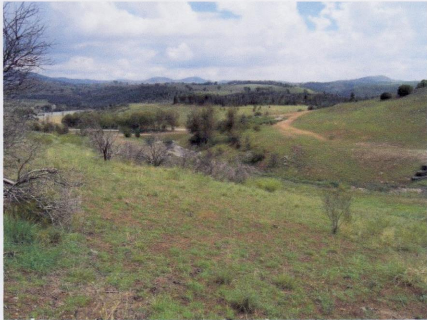
Spillway at LMWQCC
