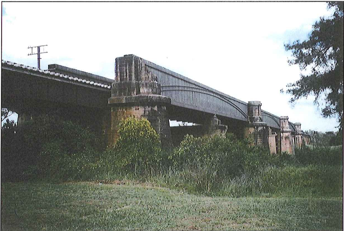
Figure 7 – Menangle Railway Bridge, March 1999
