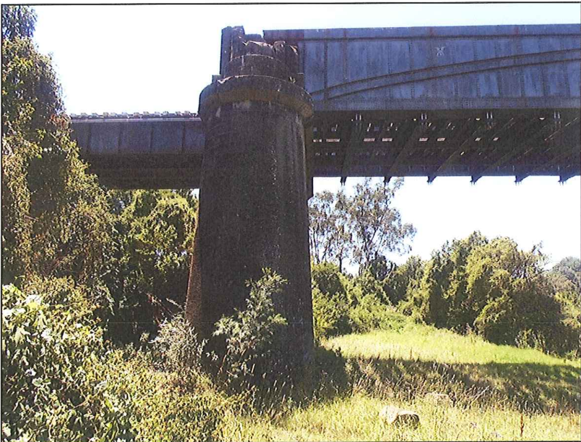
Figure 10 – Northernmost Sandstone Pier of Menangle Railway Bridge, December 2012
