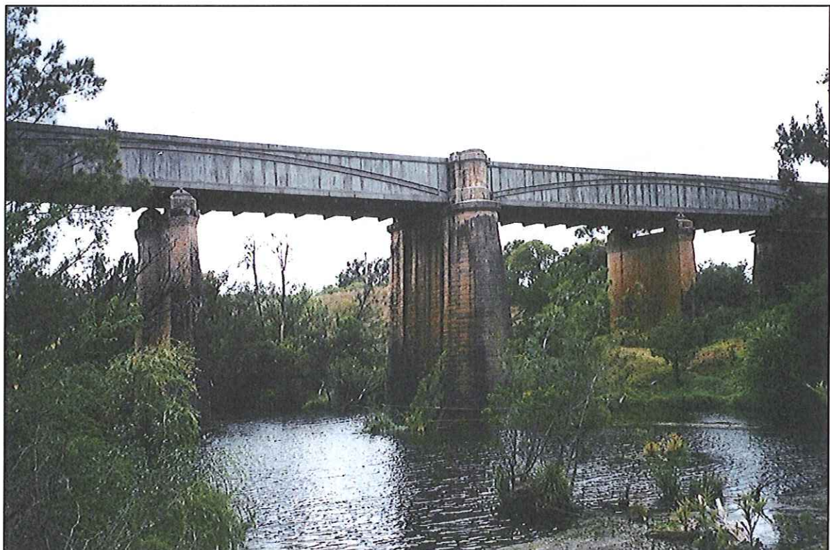
Figure 8 – Menangle Railway Bridge, February 2003
