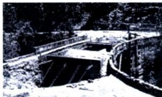
Figure 8 The arch exposed and old fill removed. (DPW&S)
