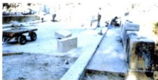
Figure 9 (left) The concrete road slab covering the stone arch (Henry Kullas) and (right) The restored bridge. It looks, to all intents and purposes, to be the original structure (DPW&S). However, the stonework is a façade with a load-bearing bridge inside.
