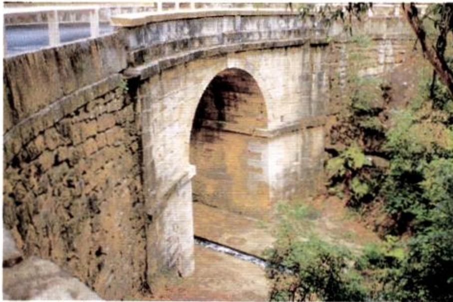
The 1833 Lennox's Horseshoe Bridge over Lapstone Creek, is the oldest surviving bridge on the Australian mainland.
