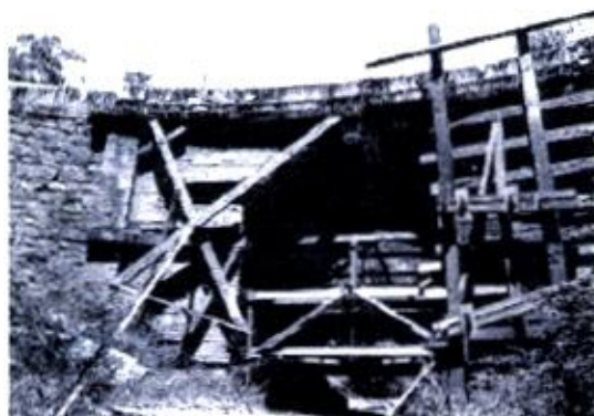
Figure 7 Temporary support of stonework. (DPW&S)
