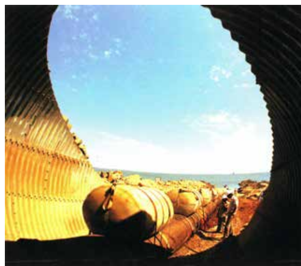
Figure 11: Trunkline 1 under construction
