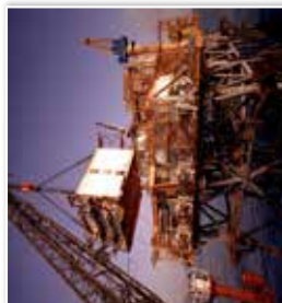
North Rankin platform under construction
