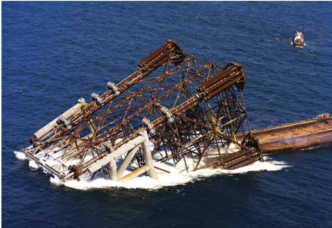
Figure 10: NRA Platform jacket being lowered
