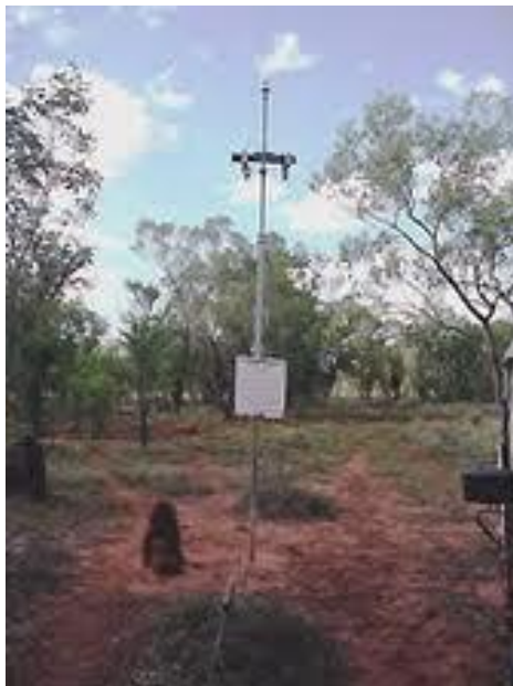
One of the Oppenheimer poles in the preserved old line section near the “joining point”.
