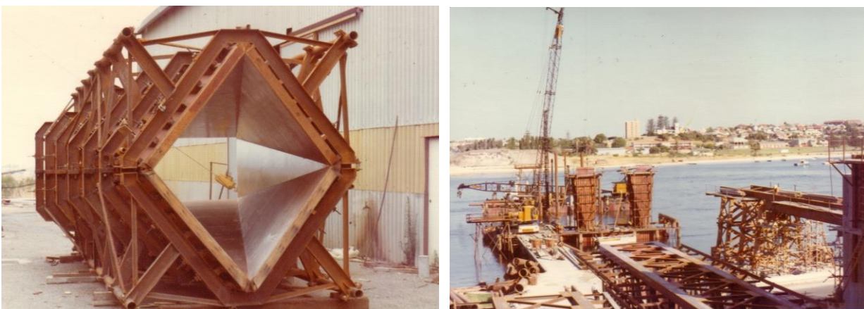
Figure 8. Left: Steel pier column forms; Right: Placing the forms on the pile cap (Photos J O Clough & Son)
