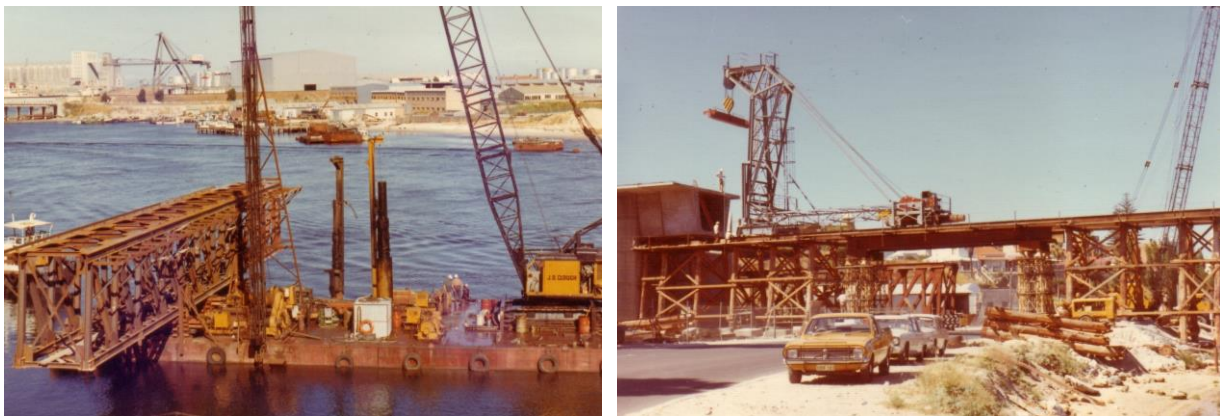
Figure 10. Left: Truss section being moved into place by crane barge; Right: South shore span falsework with placing gantry in position (Photos J O Clough & Son)
