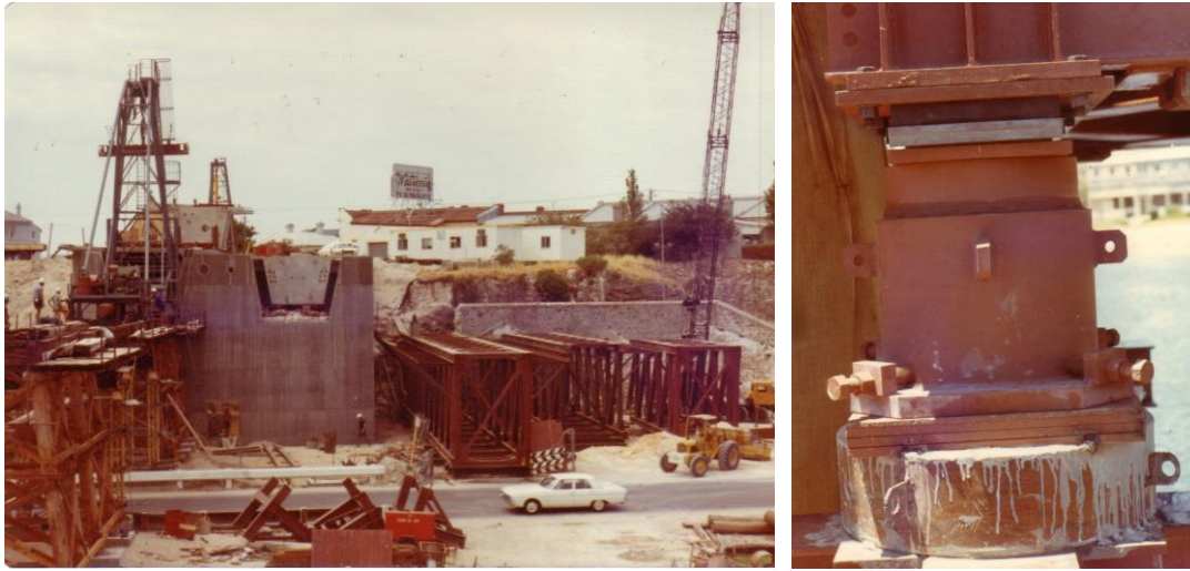
Figure 9. Left: Assembly of falsework trusses on south bank; Right: 200t capacity sand jack (Photos J O Clough & Son)
