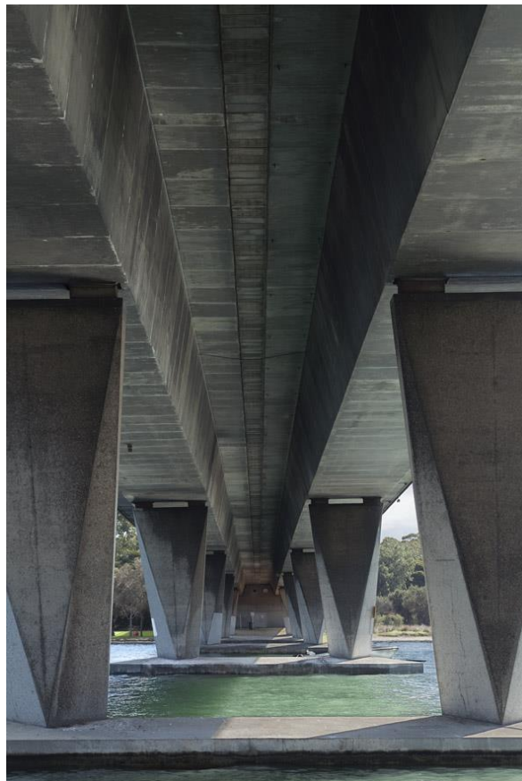
Figure 5. View of the underside of Stirling Bridge looking north. The view highlights the clean lines of the bridge beams and the architectural profile of the columns (Photo Anthony Riddette)
