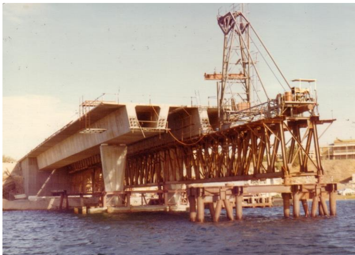
Figure 12. Stage 1 upstream row completed, downstream row placed but not yet stressed. (Photos J O Clough & Son)
