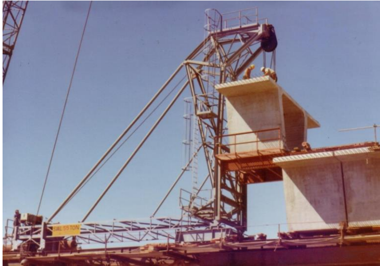
Figure 11. Unit transporter connected to placing gantry prior to lifting (Photo J O Clough & Son)
