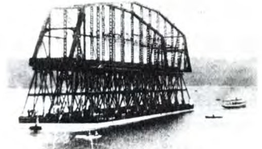
Truss floating in mid-stream
