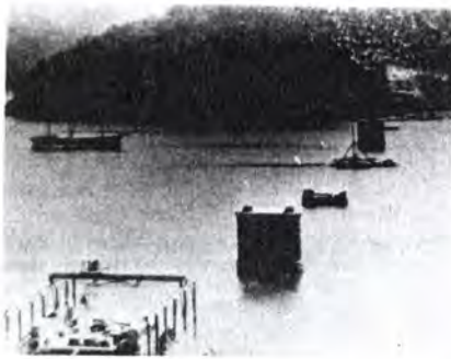
Foundations, piers 1 and 4 complete
