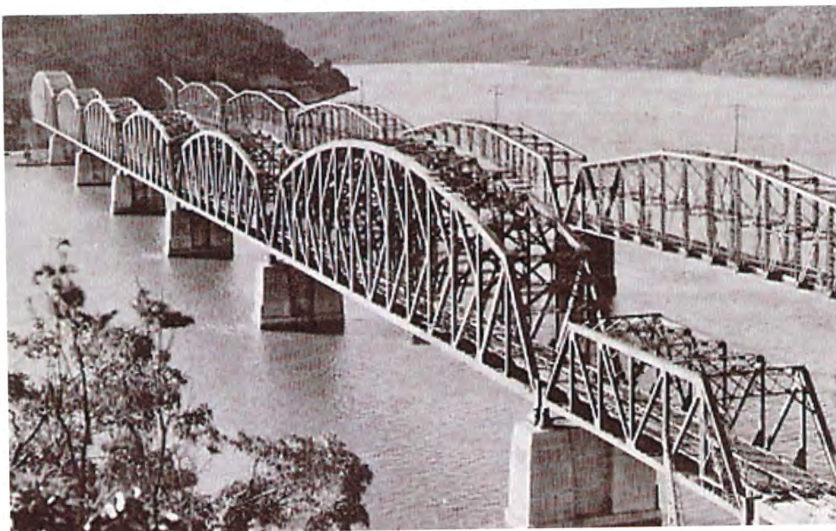
1946 bridge, left, still in service, 1889 bridge right, demolished.
