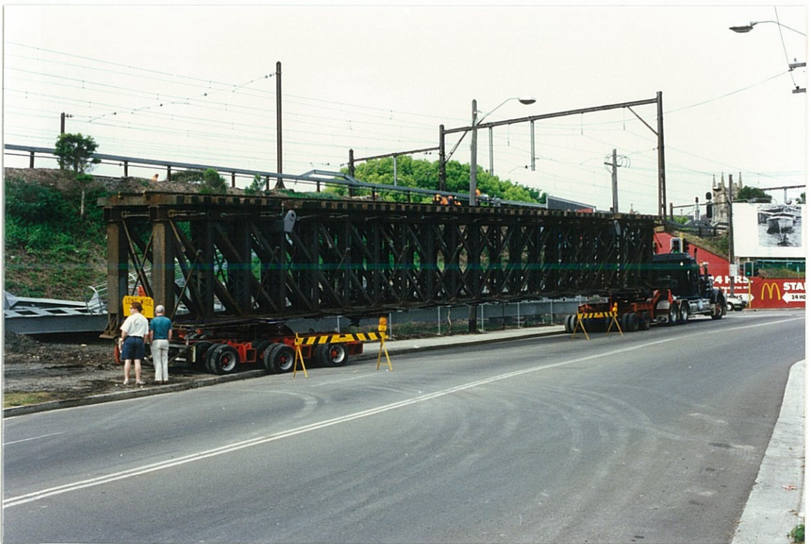
The surplus Whipple trusses were taken to St Marys and stored for future use.
