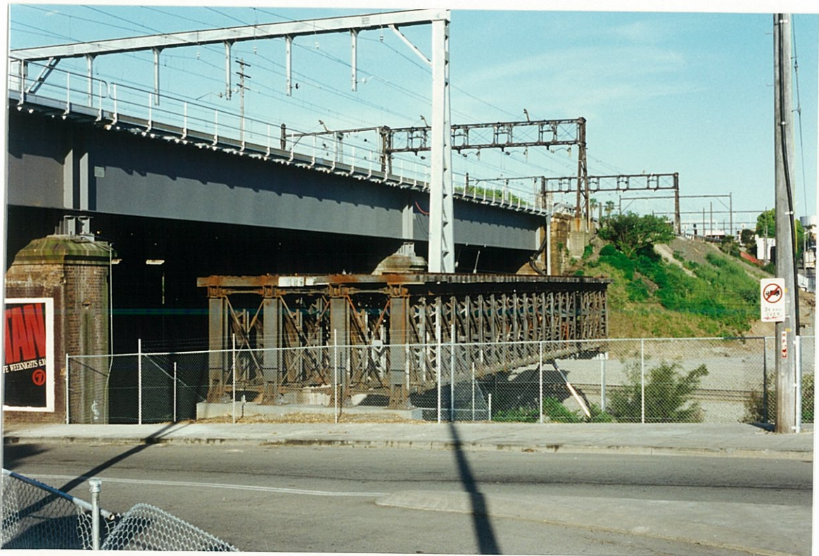
The completed project, the new plate web girder viaduct and two Whipple trusses on permanent display. The last photograph suggests the HEM plaque could be attached to the 1886 brick pier or to an end post of one of the trusses.
