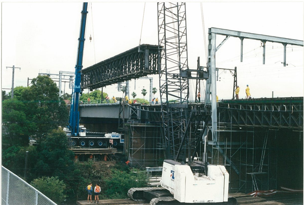
A Whipple trusses being lifted out of position, 2nd October, 1993
