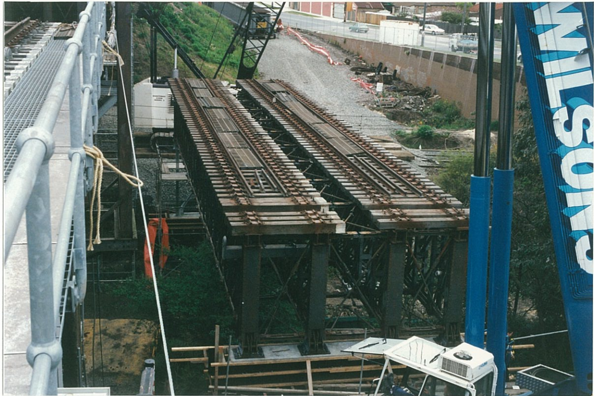
Both display trusses in position over Long Cove Creek.
