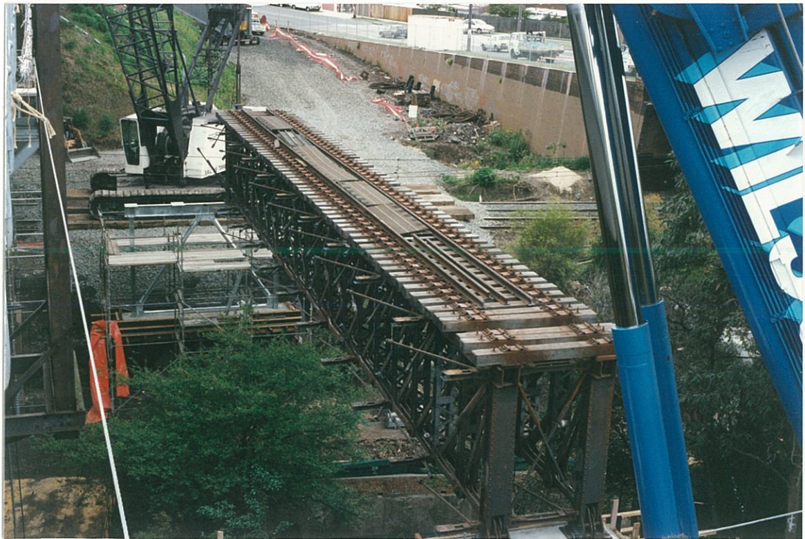
The first of the display trusses on its supports.
