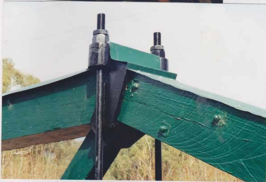
McKanes Bridge, the hip joint and shear rods in the McDonald timber truss. Note the pair of rods outside the main timbers and the cast iron joint shoe.
