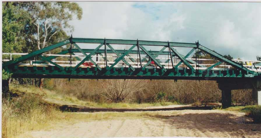
General view of the bridge and a typical McDonald truss span.
