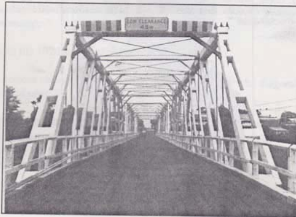
Figure 2.3.4f – Morpeth Bridge. The oldest serving overhead timber truss bridge recently celebrated its centenary (opened 1898).
