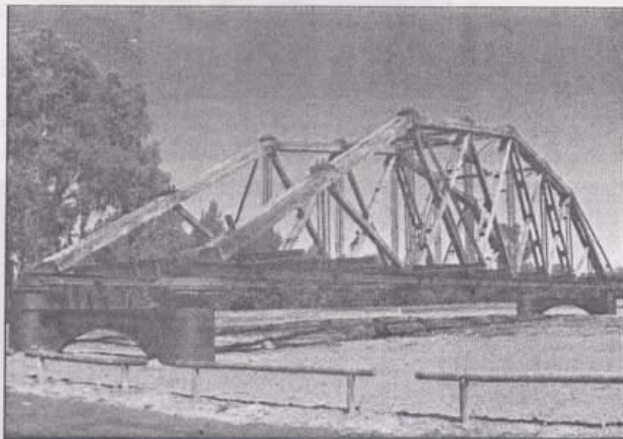
Figure 2.3.3i – A span of the original Lachlan River Bridge at Cowra on display at a nearby riverside park. The bridge utilised steel tension members and timber compression members in an early example of composite design.
