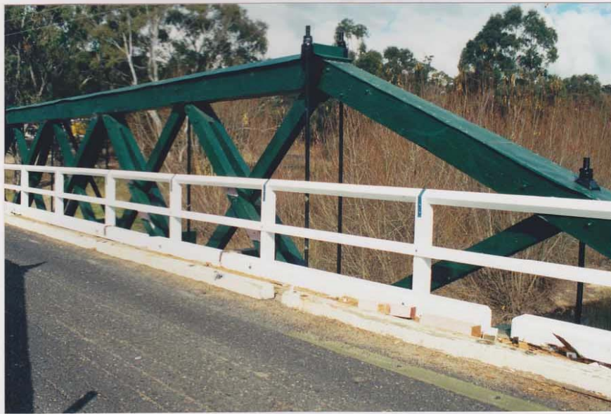
McKane's Bridge, end portion of a McDonald truss and one of the stone abutments, and an interior view of the bridge.
