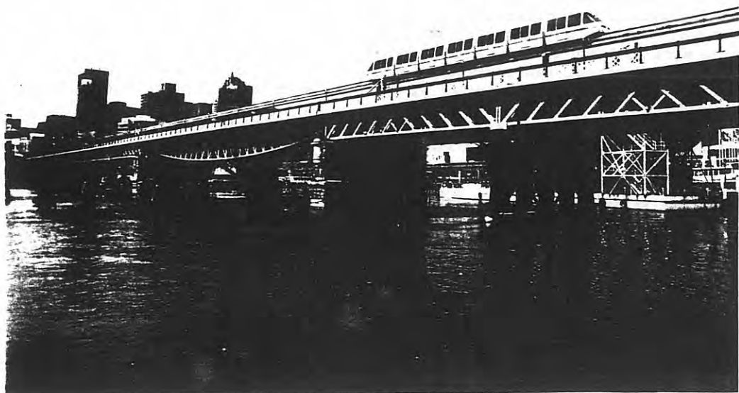
The finished bridge
