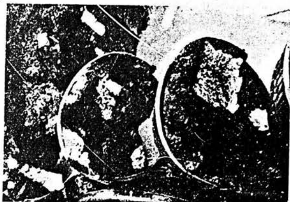
Newstead Dredge.—The dredge buckets are stripping overburden which is tipped on to the resoling stacker in this almost dry state.
