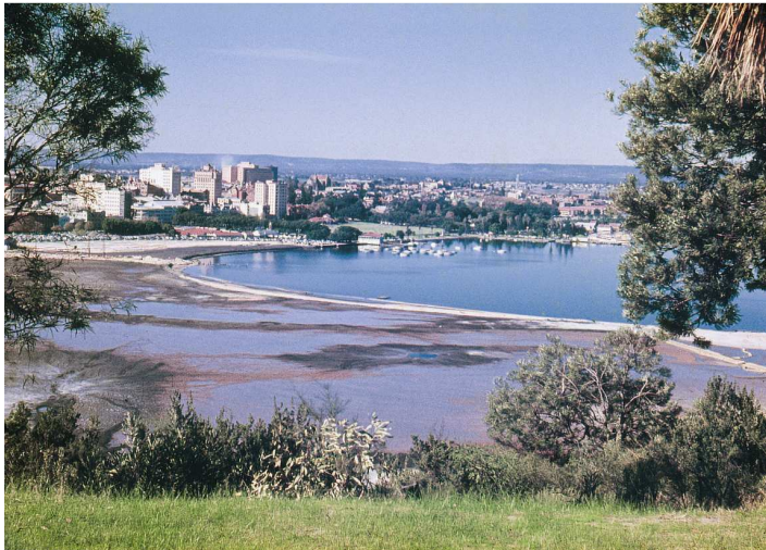
The Narrows Interchange site ca 1956
