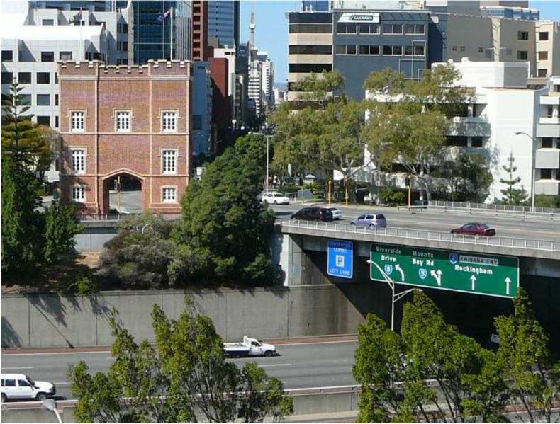
Barracks Arch and Malcolm Street Bridge over central section of freeway
