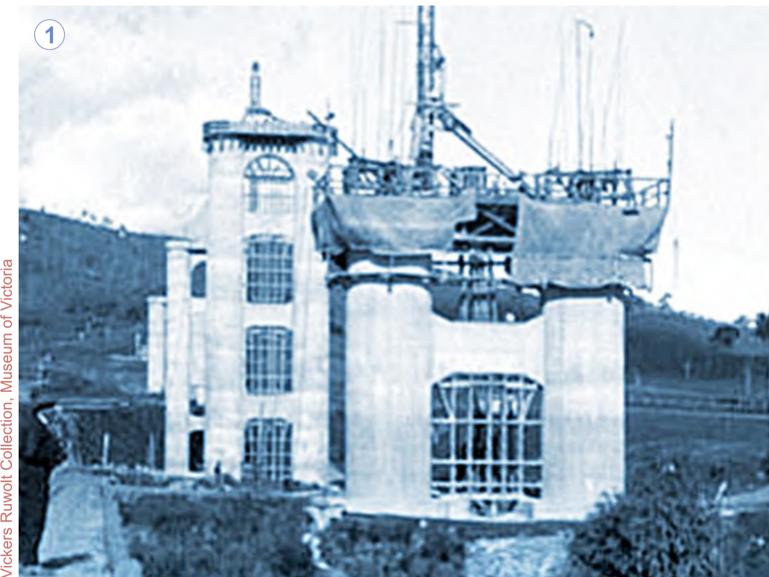
1. Building the concrete towers with movable formwork 2. One of the trusses assembled at the Ruwolt factory 3. Working from the temporary platform
