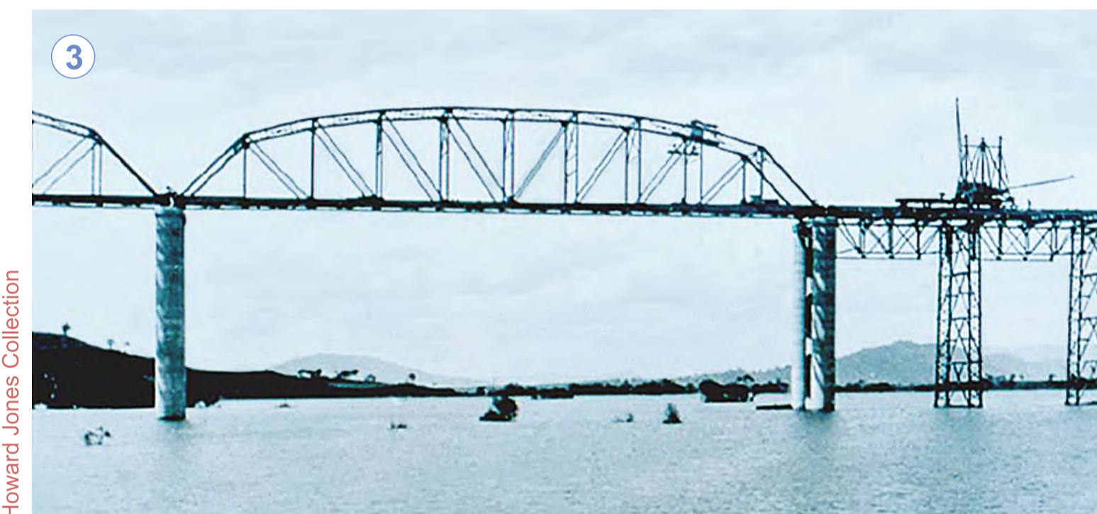
1. Building the concrete towers with movable formwork 2. One of the trusses assembled at the Ruwolt factory 3. Working from the temporary platform
