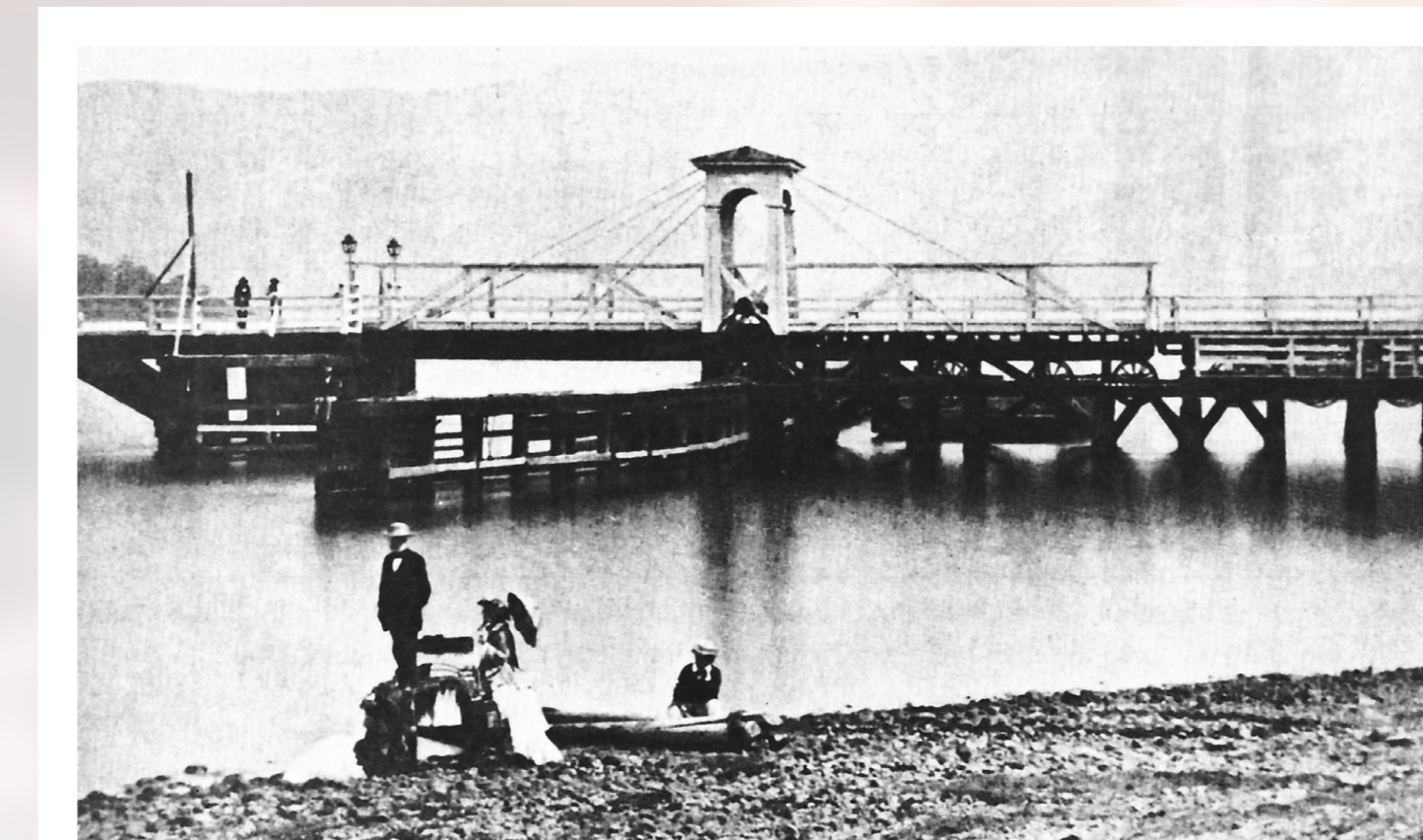
Bridge No.1 view downstream on the northern banks showing tower and timber tow path for vessels. The iron wheels are visible on the right side of the tower. – Courtesy Tasmanian Archives and Heritage Office [TAHO]
