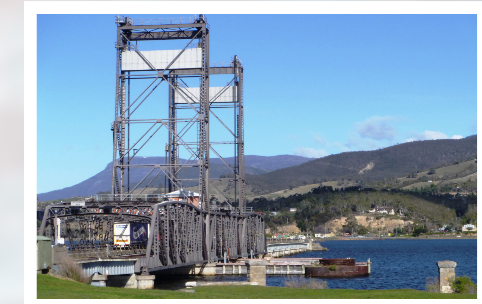
Bridge no.4 the current bridge looking south shows heritage items of the early abutments and steel caisson of the 1893 bridge. On the southern bank is the quarry where stone was dug with pick and shovel and barrowed to the water's edge – Courtesy Ian D Cooper
