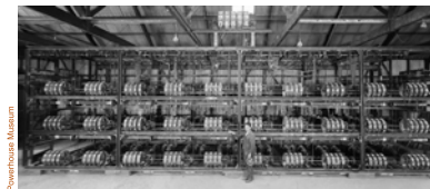
Two of the indicator drive and adding machine modules
