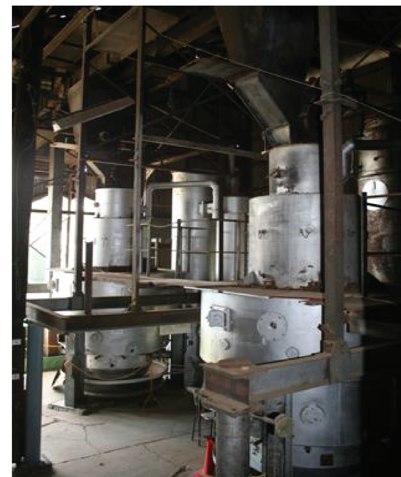
Coal Fired Gas Producers Nos 1 & 2 - 1952
