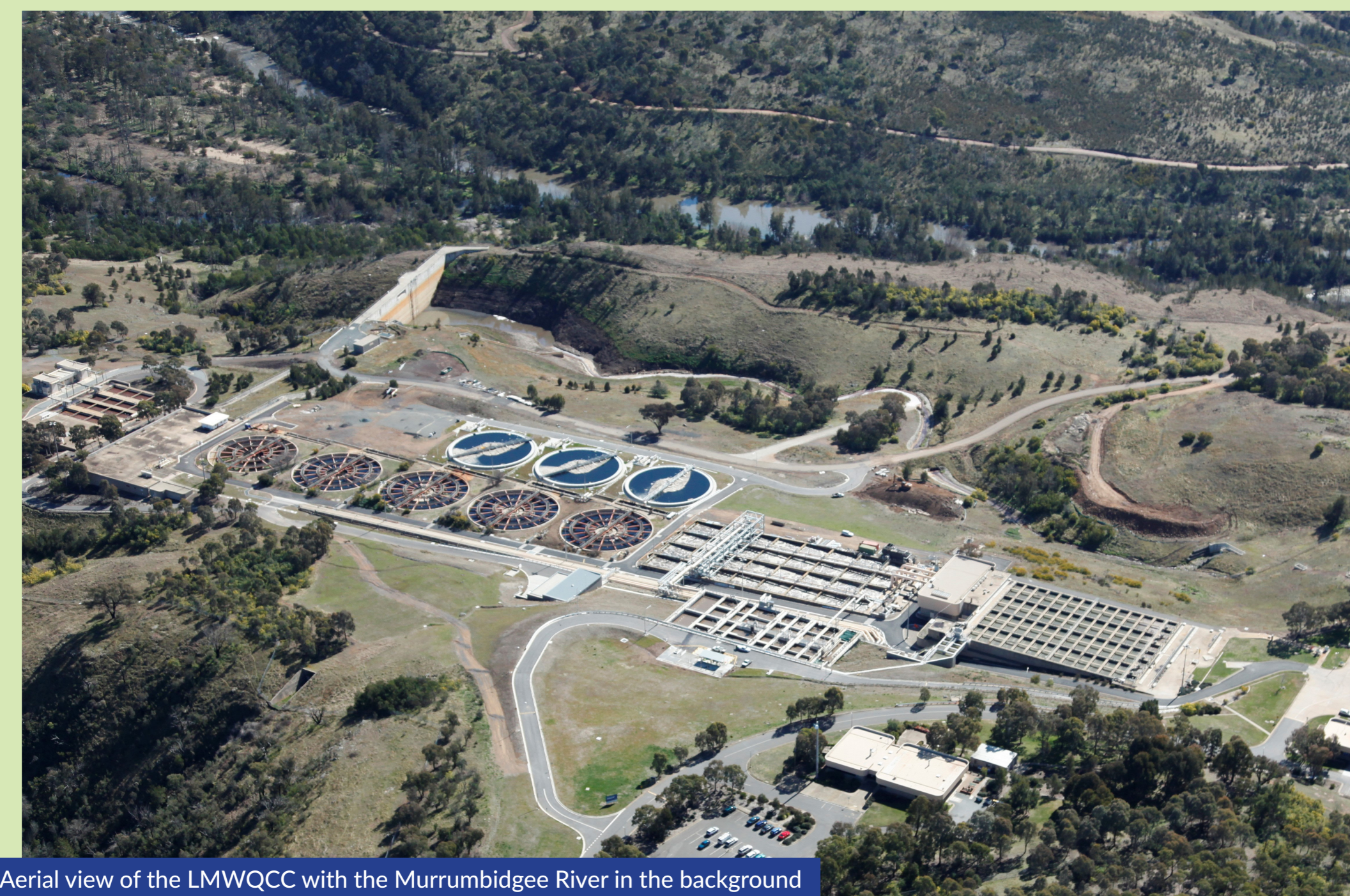
Aerial view of the LMWQCC with the Murrumbidgee River in the background
