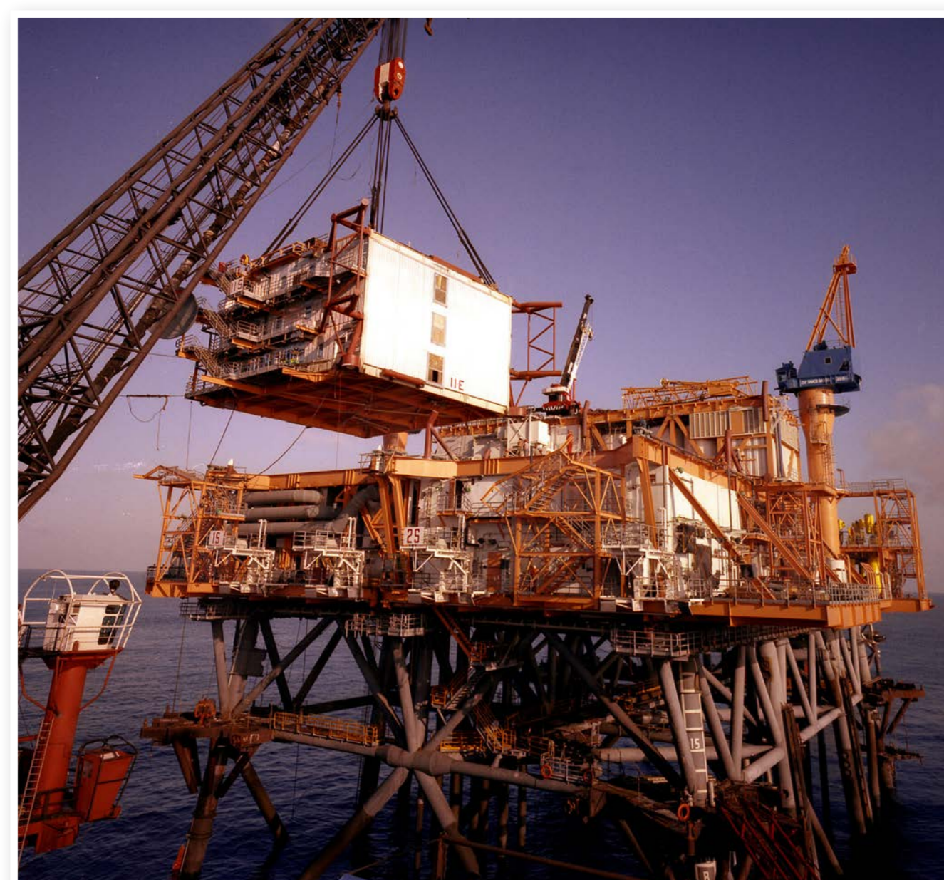
North Rankin platform under construction
