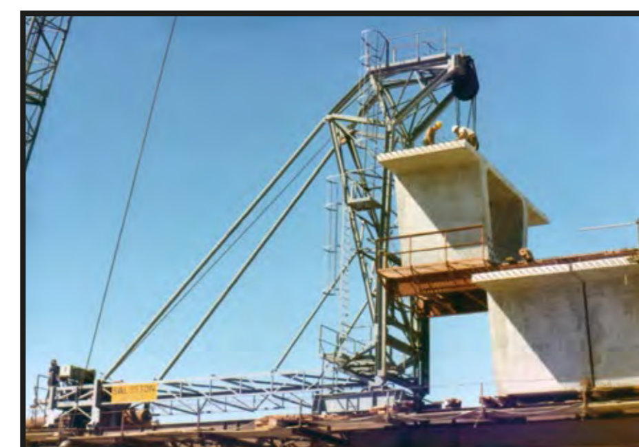
Gantry crane placing a concrete beam unit onto falsework
