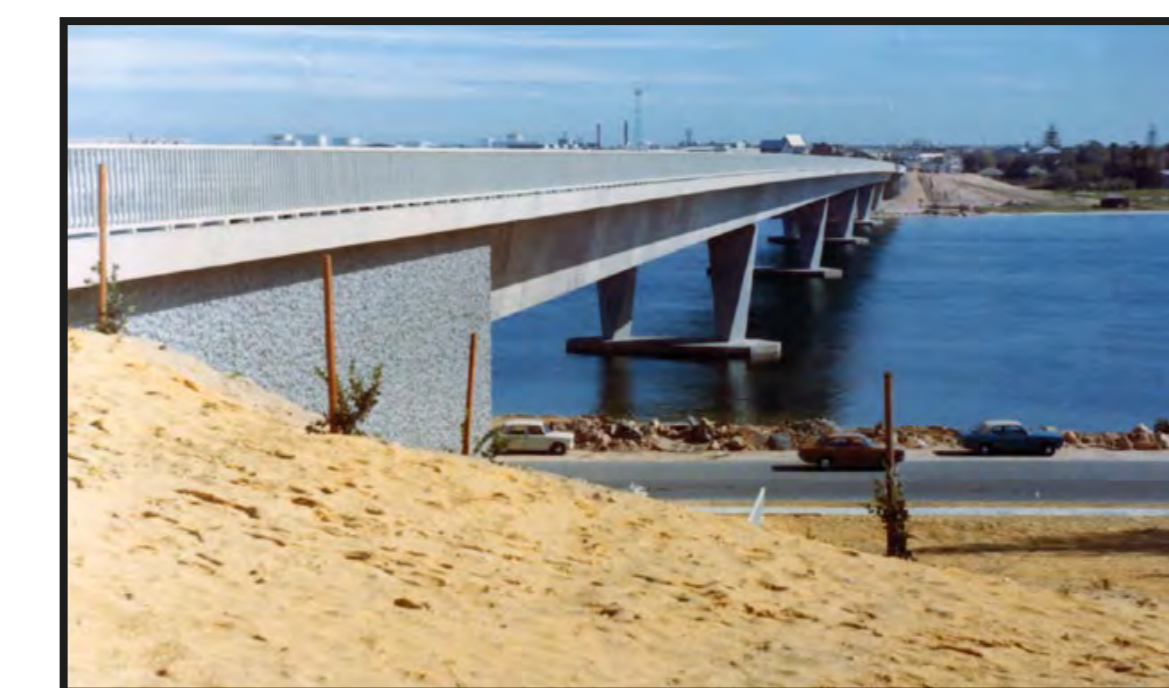
View of completed bridge from south abutment, May 1974
