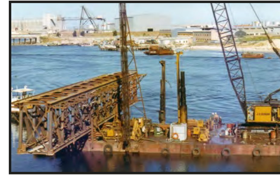
The crane barge used to drive piles and transport the steel falsework
