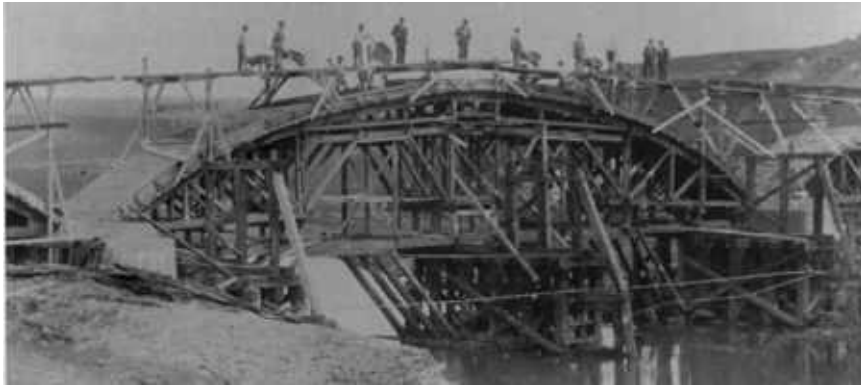
Placing concrete in the central span 1899. Image: University of Melbourne Archives
