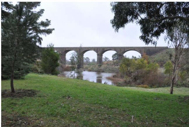
Malsbury bluestone viaduct is still an impressive structure today
