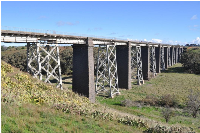
Moorabool Viaduct today carries a national standard gauge track
