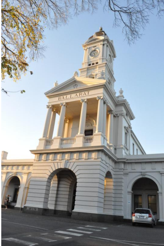
The imposing entrance to Ballarat Railway Station
