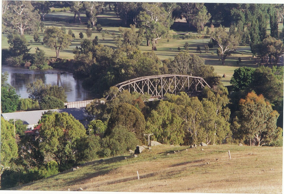
The historic bridges as they cross the Murrumbidgee River flood plain at Gundagai. Top - in the foreground is the the road crossing, 1867 iron truss road bridge, the Prince Alfred Bridge, and the long timber girder viaduct. In the middle is the long timber truss railway viaduct. Bottom - the 200-foot steel railway truss that carried the Tumut line over the river.
