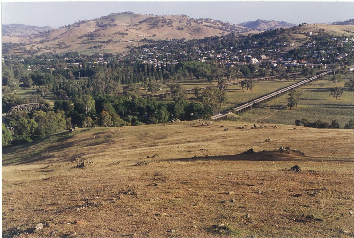
The two sites of historic Gundagai. Top - the layout of the first town on the flood plain of the Murrumbidgee River which the flood of 23 June 1852 swept away. The new town was sited on the southern slopes of Mount Parnassus, as shown in the bottom photograph. Consequently, the decks of the 1867 road and 1903 rail crossings were built above the maximum flood level.
