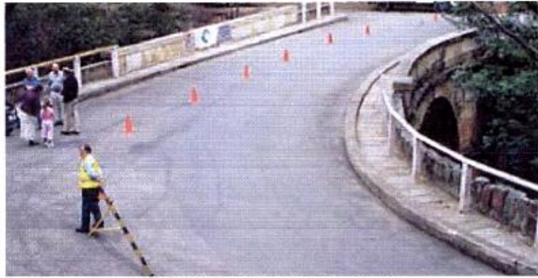
The site on Horseshoe Bridge
