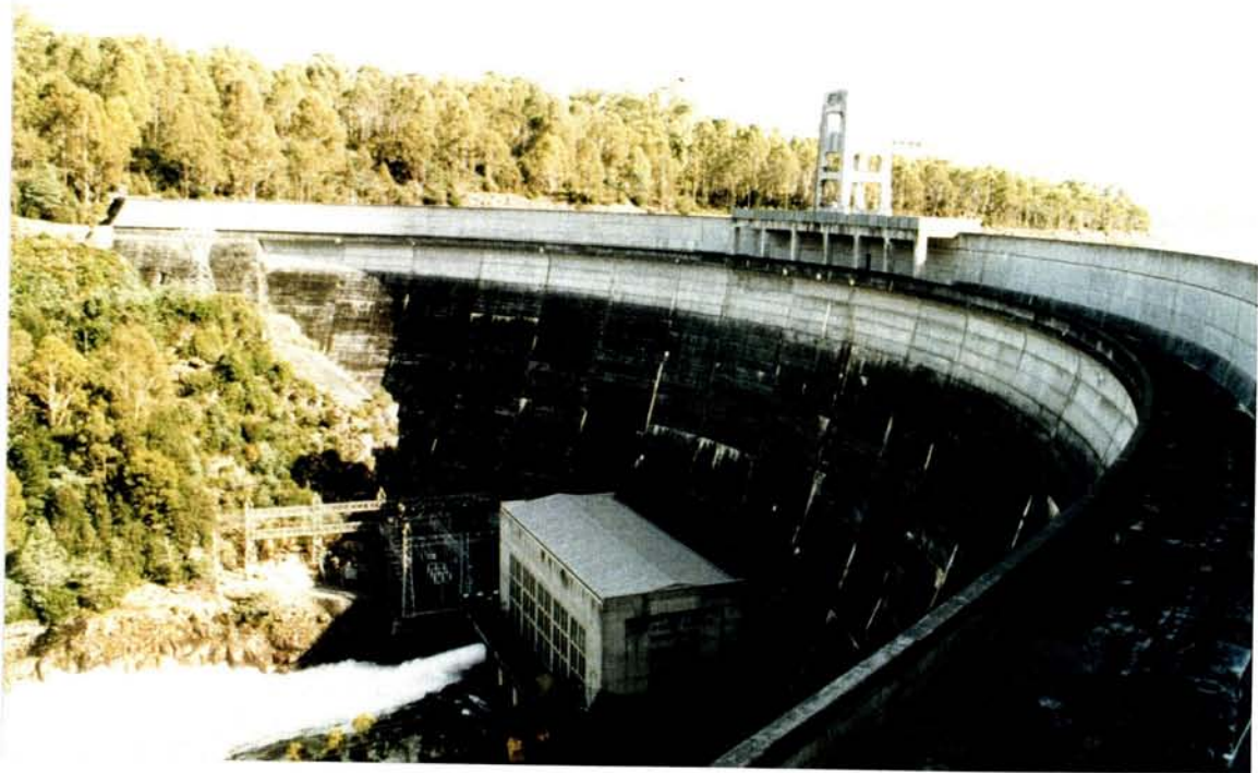
Fig.12 Clark Dam and Butlers Gorge Power Station
