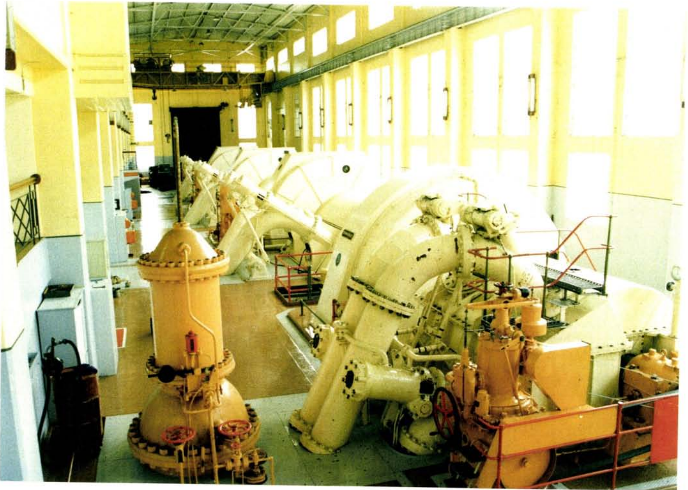
Fig.9 Boving 3 Jet Machine
