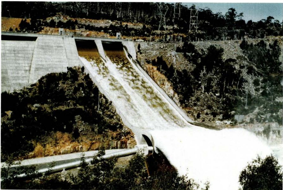
Fig.13 Butlers Gorge Spillway
