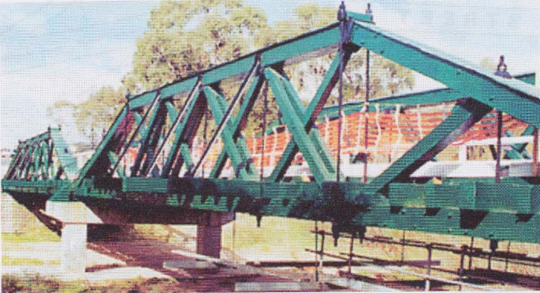
The two McDonald Truss spans of McKanes bridge and below the standard drawing of a 90 foot McDonald Truss.
