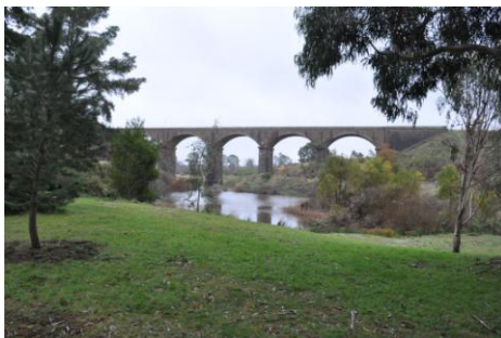
Malmsbury Viaduct Image: Owen Peake
