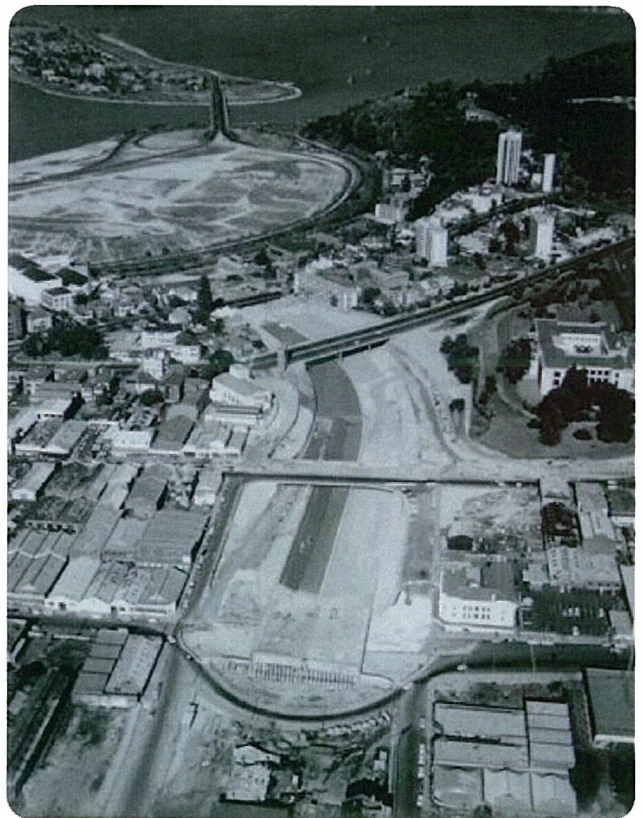
Central Section under construction in 1968
